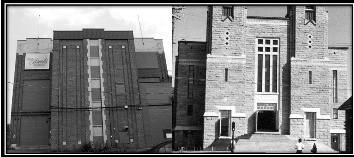
Figure 29. False pediment façades. (Left) T. Pringle & Sons' factory. Photograph 2011, Caroline Beaudoin. (Right) Sainte-Marguerite's church. Photograph c.1950s, Fondation du patrimoine religieux du Québec, inventaire des lieux de culte du Québec 2003-05-039-57-01.
