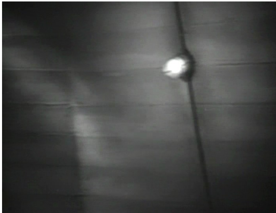
Fig. 3.4 The horizontal lines in the underground corridor
