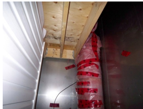
b) Insulated pipe transports the supply and return air
