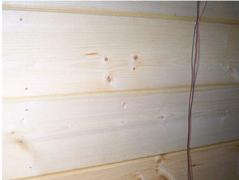
Fig. 4.3 Joints between wood panels were sealed with elastomeric latex sealant.
