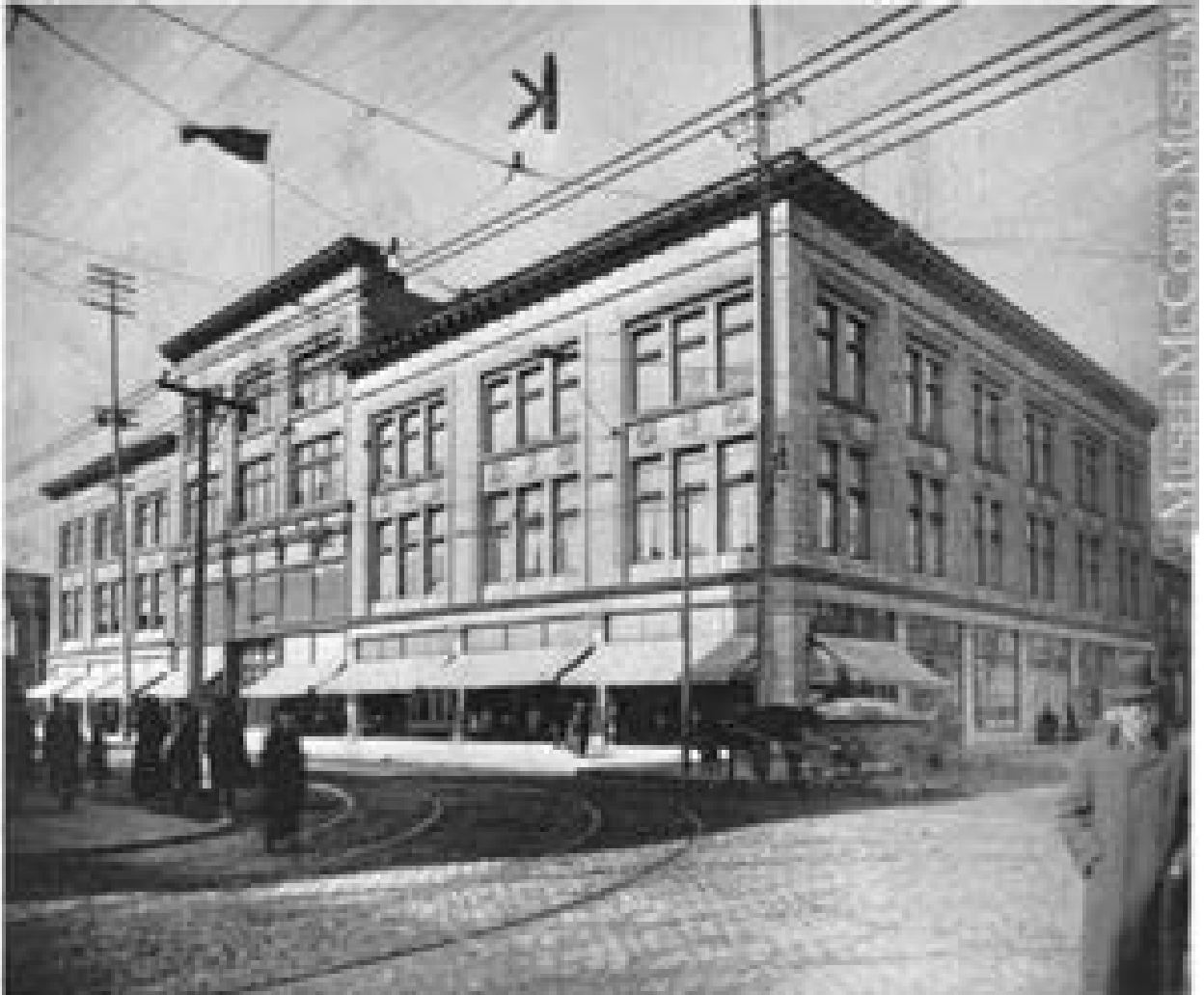
Figure 5 Goodwin's department store (future site of T. Eaton Co.), Ste-Catherine Street Montréal, QC, ca. 1912. Photographer unknown. c. 1912. Silver salts on paper, gelatin silver process. Source: McCord Museum.
