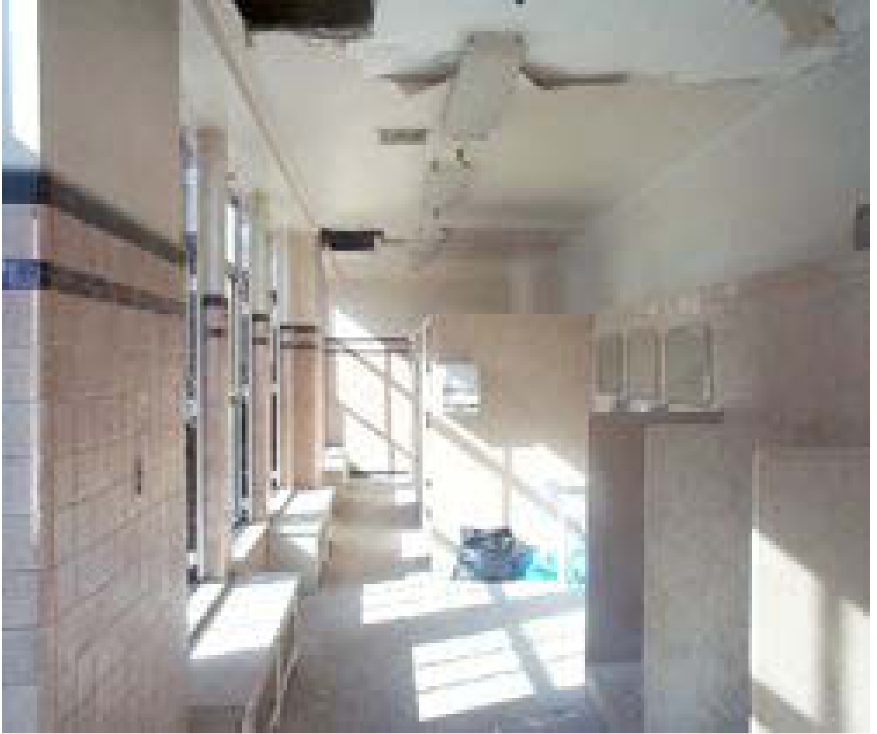
Figure 4 Ninth floor men's public washroom. c. 2002 Photograph. Source: Urban Explorers Montreal intervention. The 9th Floor . Urban Explorers Montréal, n.d. Web. Accessed 22 Nov. 2009.
