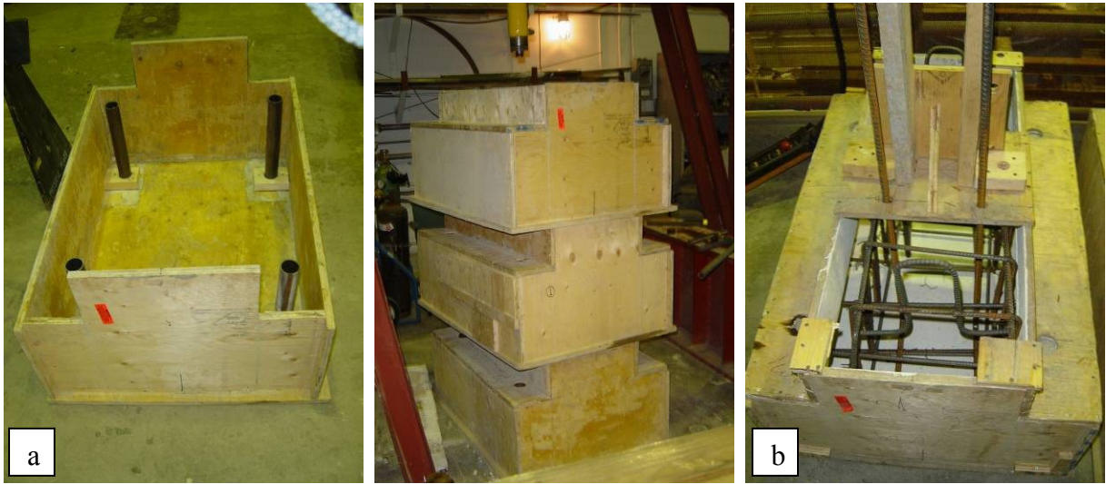
Figure 3.11: (a) Prepared wood forms for concrete footings, (b) Steel reinforcement inside the RC footings
