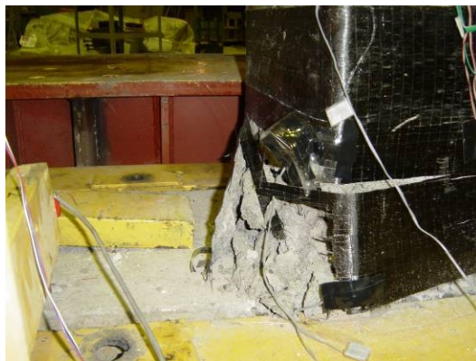
Figure 3.21: Observed ultimate failure for column RMC-CW-1S by FRP rupture and crushing of concrete masonry
