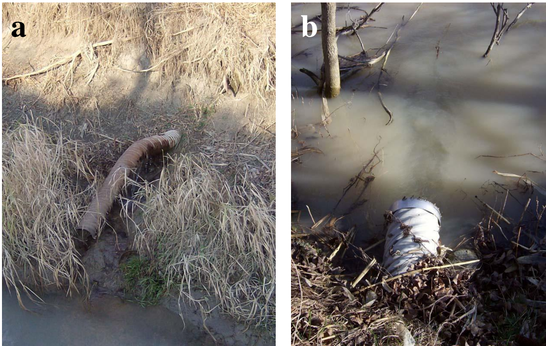
Figure 3.11. (a) Exposed drainage pipe end #7 is vulnerable to flow and ice due to acute bank erosion. (b) Water draining from pipe end #29 on 28 November 2009 and being more transparent than stream flow, thus indicating lower suspended load.
