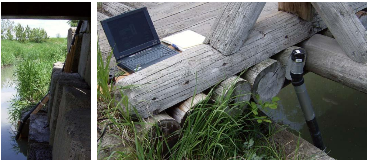
Figure 2.4. Setup of the pressure transducer on a privately-owned bridge (Figure 2.1b).
