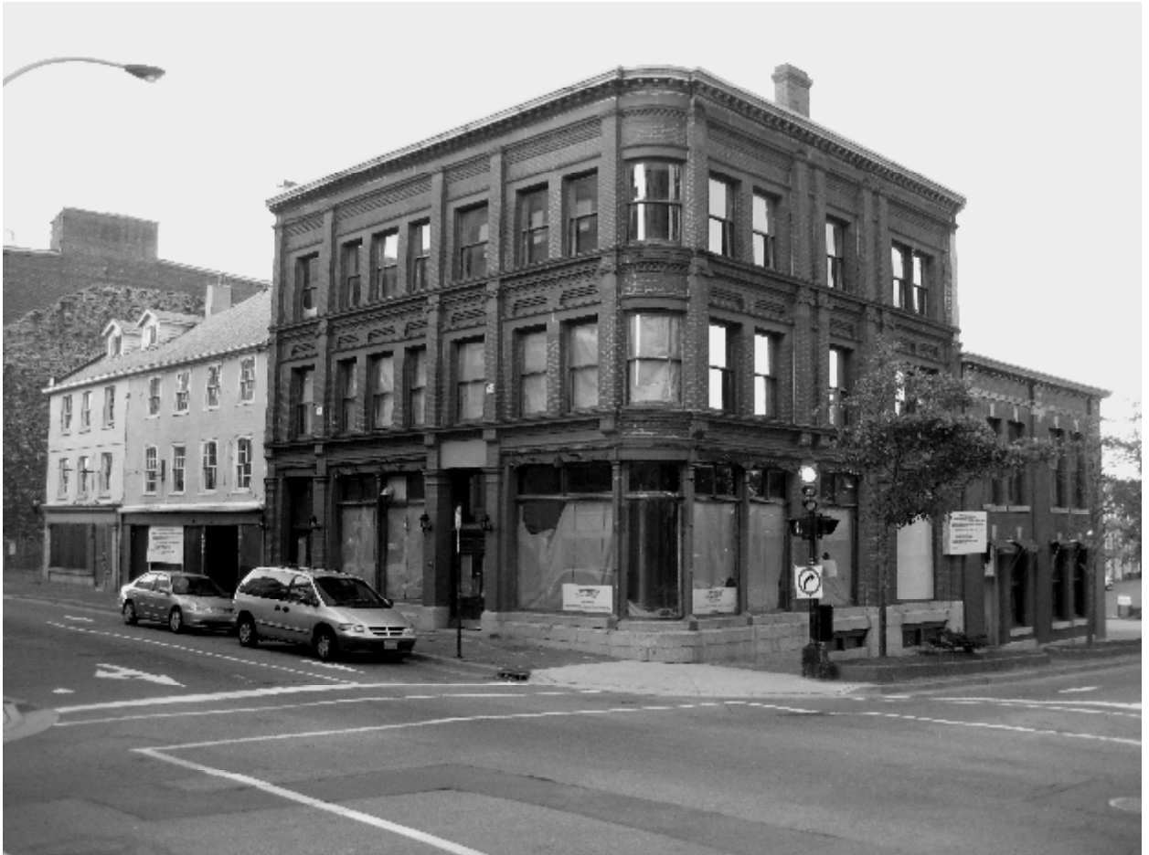
Figure 5: View of buildings from the corner of Hollis and Duke Streets. Left , Harrington and Fishwick Buildings; centre , the Shaw Building; right , the south side of the Imperial Oil Building.
