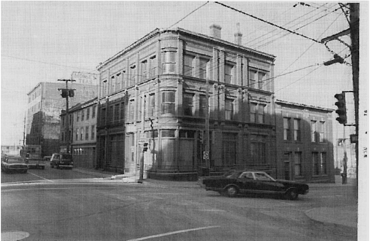
Figure 30: Photograph of buildings from the corner of Hollis and Duke Streets. Left , Harrington and Fishwick Buildings; centre , the Shaw Building; right , the south side of the Imperial Oil Building.
