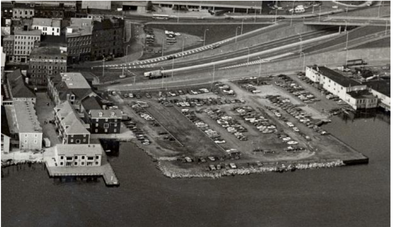
Figure 29: The Cogswell Street interchange after its completion. Without the Harbour Drive project, the interchange was downgraded to feed traffic onto Hollis Street so that drivers pass through the middle of the heritage district, with the Harrington, Fishwick, and Shaw Buildings to their left.
