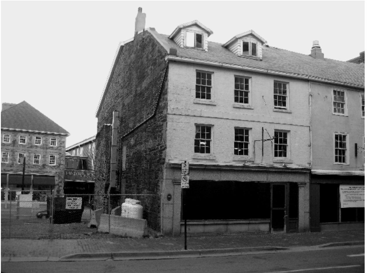
Figure 13: The Harrington MacDonald-Briggs Building, 1865 Hollis Street.
