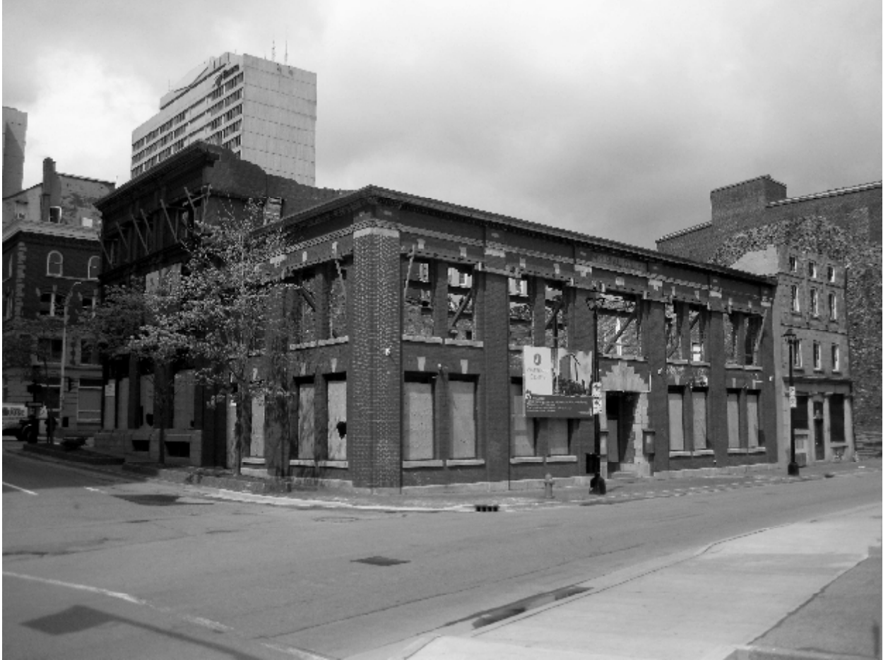
Figure 43: The buildings from Upper Water Streets. Left , south side of the Shaw Building; centre , the Imperial Oil Building; right , the Harrington Building.
