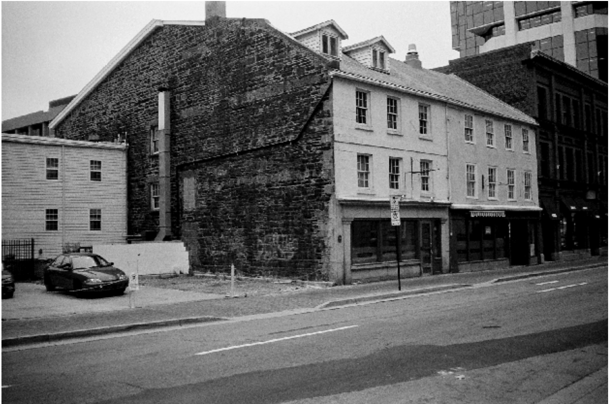
Figure 4: View of buildings on Hollis Street. Left to right , Harrington Building, Fishwick Building, and west side of Shaw Building.
