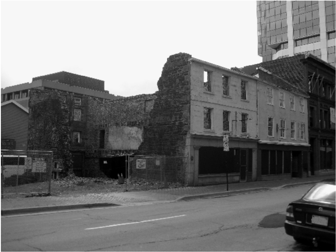
Figure 40: Remaining walls of the buildings from Hollis Street. Left , Harrington Building; centre , Fishwick Building; right , section of west side of Shaw Building.
