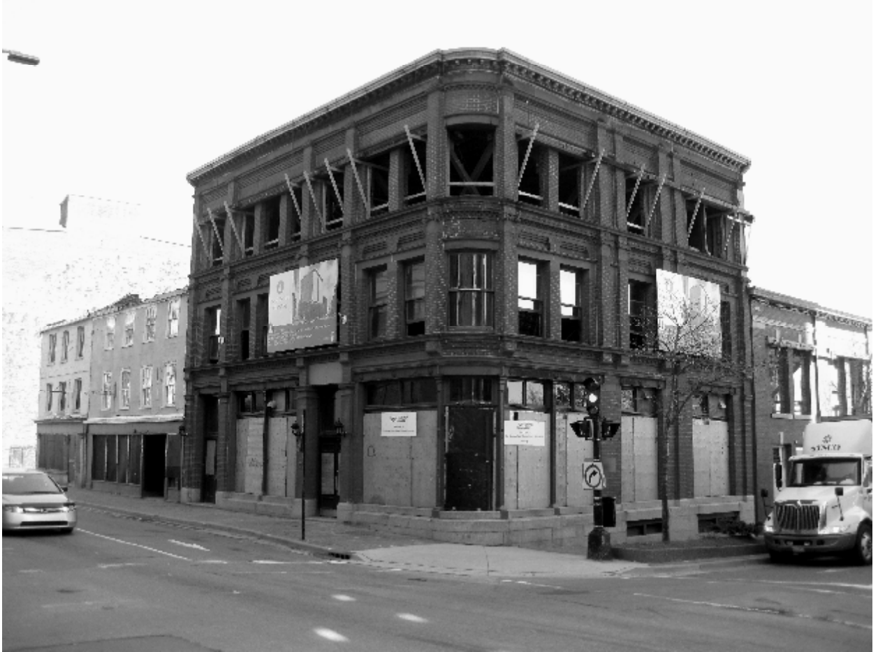
Figure 42: The buildings from the corner of Hollis and Duke Streets. Left , Harrington and Fishwick Buildings; centre , the Shaw Building; right , section of the Imperial Oil Building.
