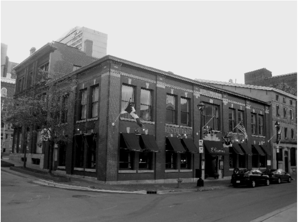
Figure 6: View of buildings on Upper Water Street. Left , south side of Shaw Building; centre , Imperial Oil Building; right , the Harrington Building.
