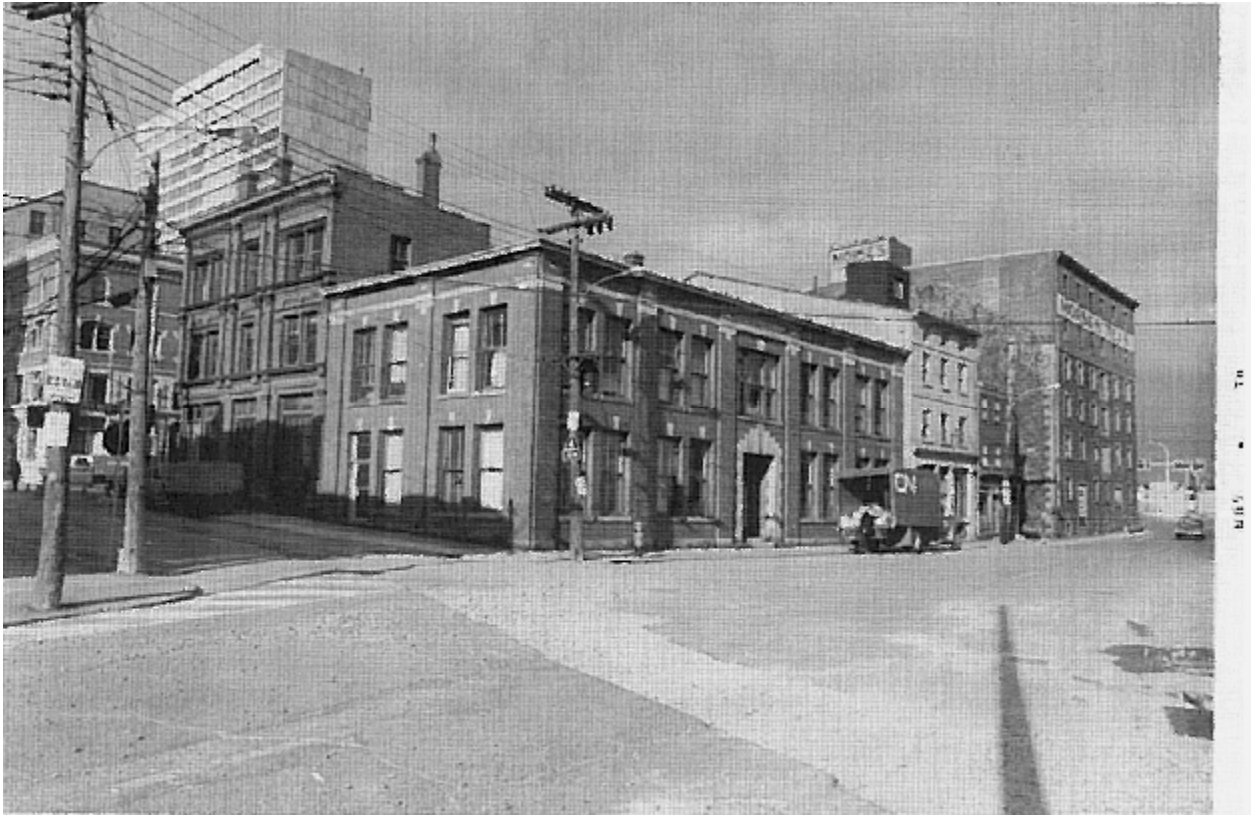
Figure 31: Photograph of buildings from Upper Water Street. Left , south side of Shaw Building; centre , Imperial Oil Building; right , Harrington and Peter Martin Buildings.
