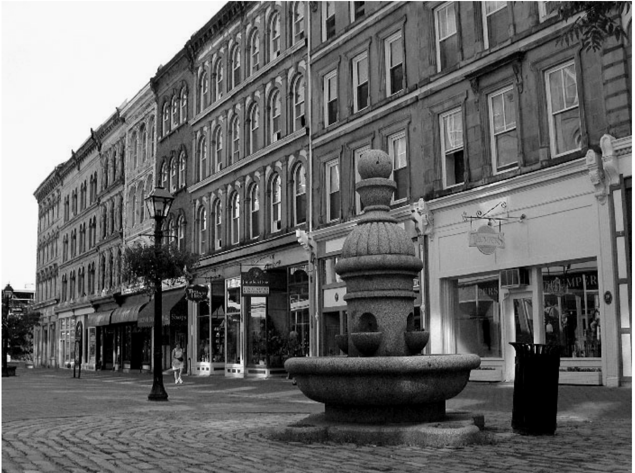
Figure 8: Granville Streetscape. Buildings occupied by NSCAD, part of Historic Properties.
