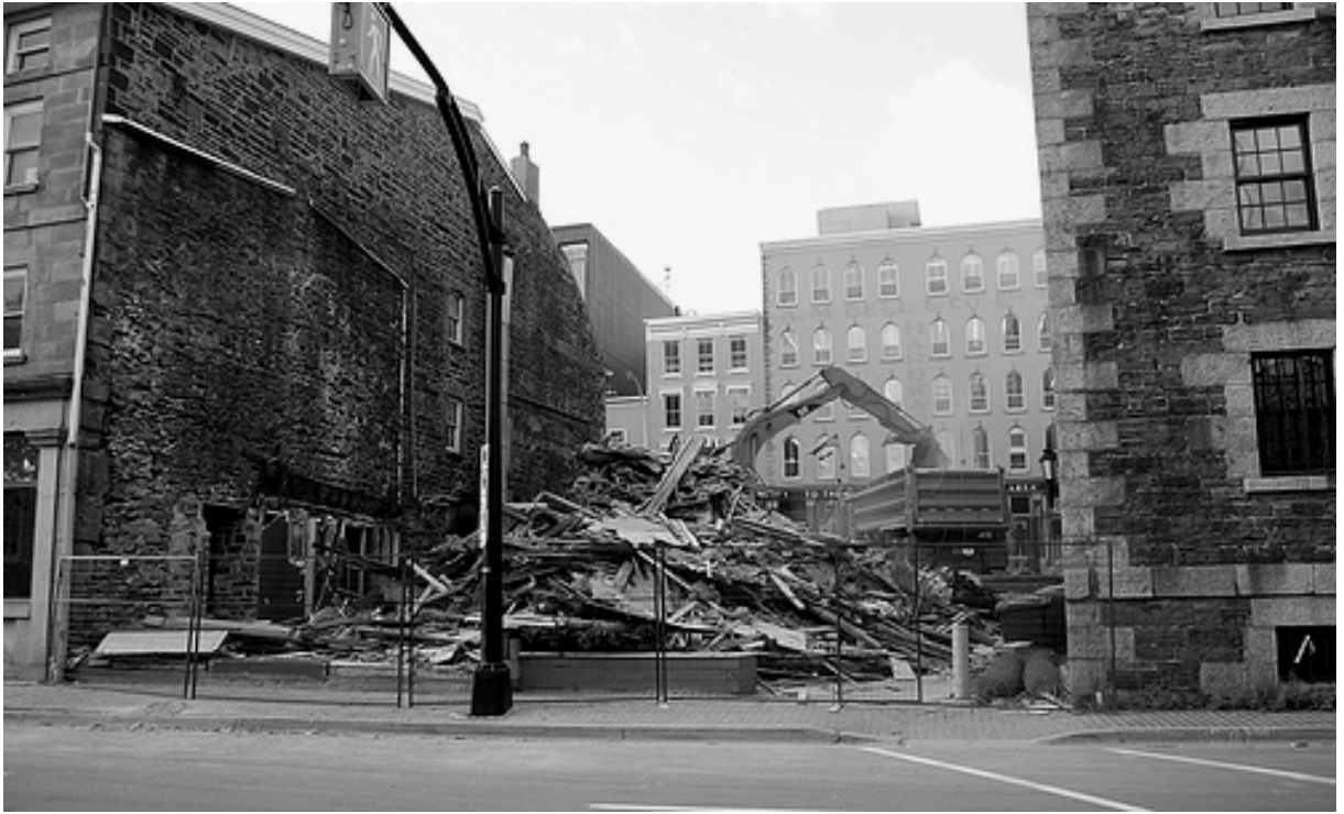
Figure 39: The demolition of the Peter Martin Liquors Building, November 2, 2008.
