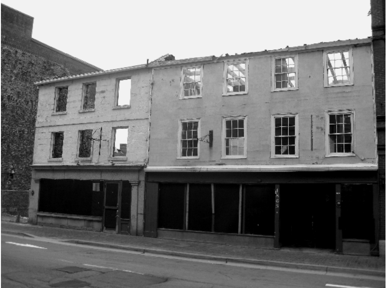
Figure 41: The Harrington Building ( left ), and the Fishwick Building ( right ).
