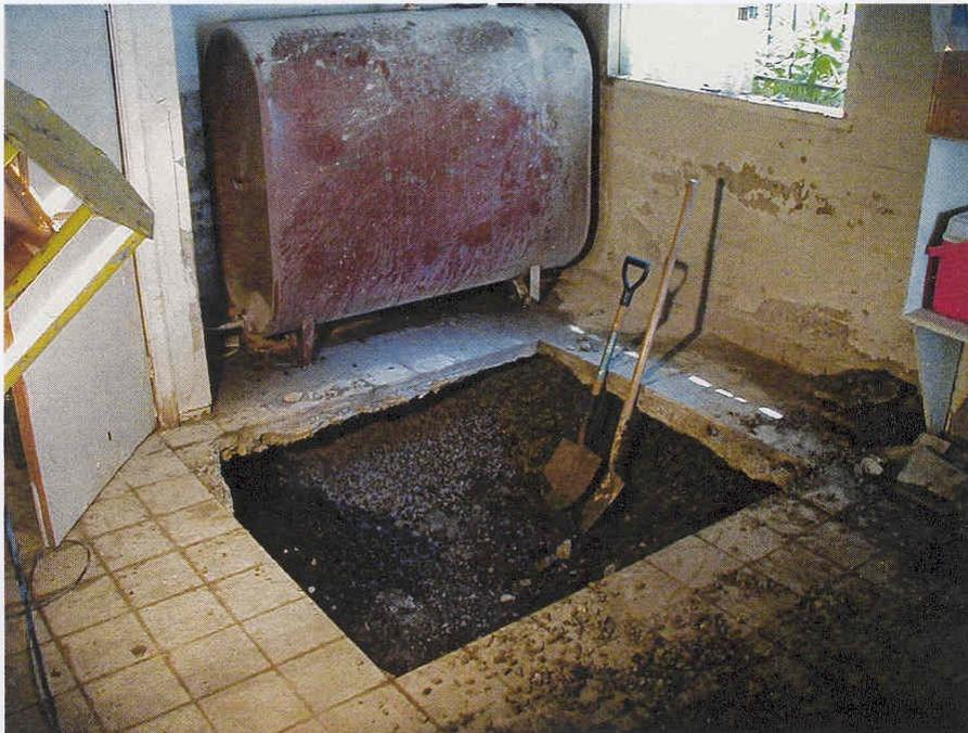
**Figure 1.3 Leaking heating oil tank and damage
