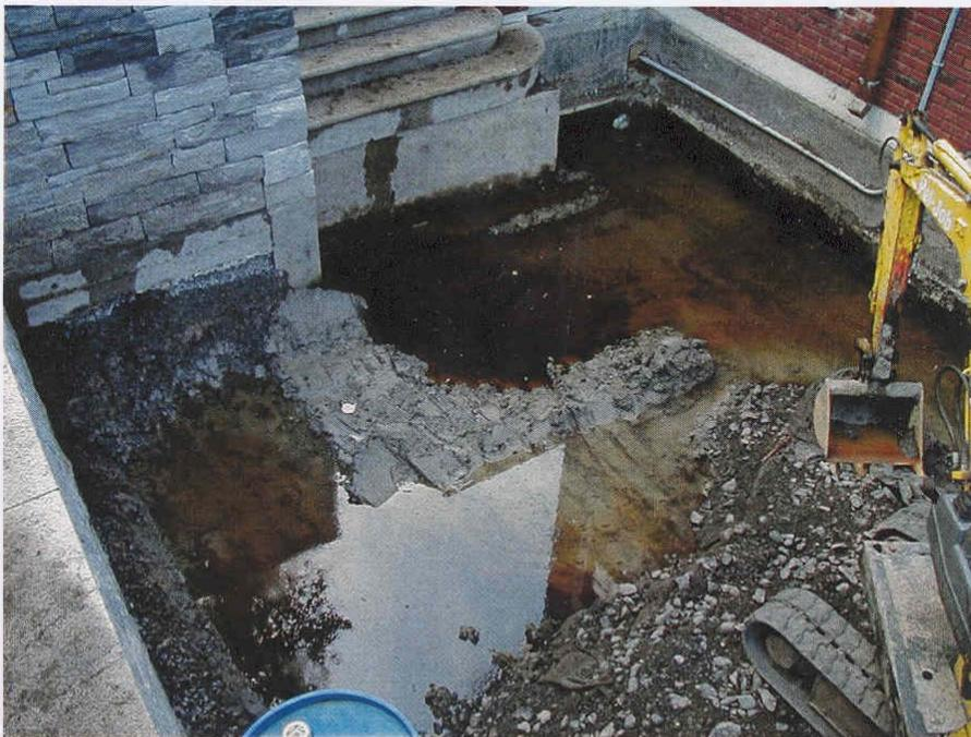
**Excavation of oil saturated gravel backfill**
