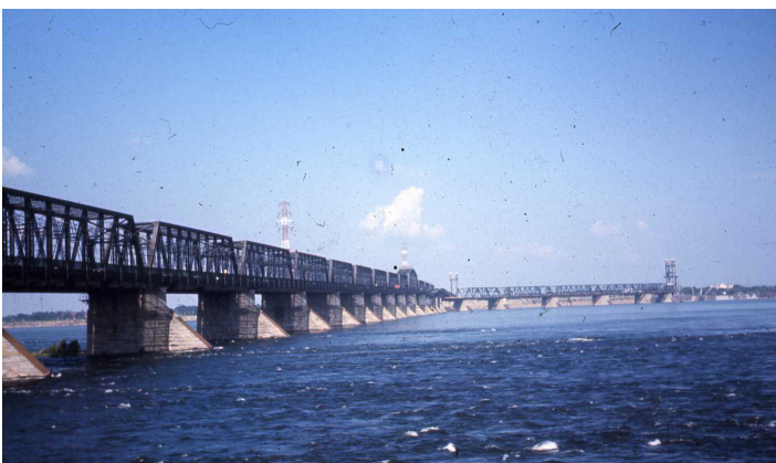
Fig. 7. Photograph (circa 1980) of the Victoria Bridge from the northwest shows the trusses rising to the higher centre span and the new spur going to the west lift-span (outlined against sky) over the seaway.
