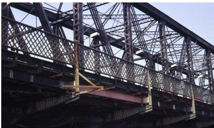
Fig. 5. Close-up view of the truss structure fabricated by riveting from narrow sheared plates, bars and angles; vertical laced girders are in compression, diagonal bars in tension. The transverse beams, attached below the truss, support the twin tracks and extended roadways.
