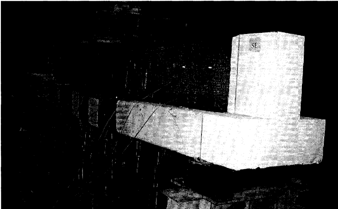
Figure 5.16 Rehabilitated girder IT-G2R at failure
