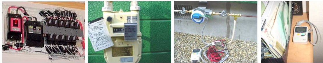
Figure 3-7 Measuring instruments (from left to right: electricity, gas, kerosene and air temperature)
