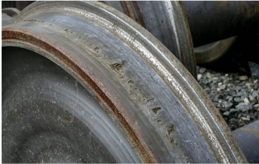
Fig. 1. 22: Wheel shelling defect.
