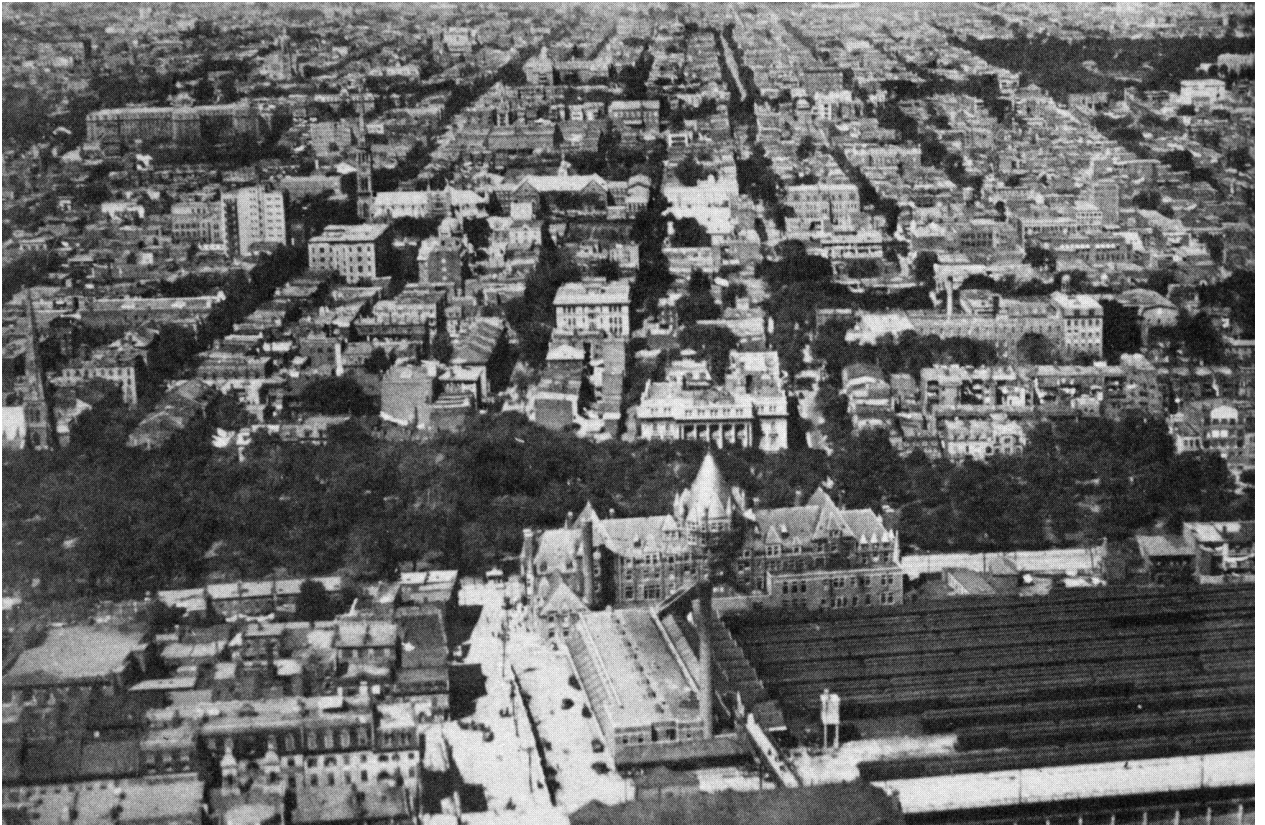
Aerial view of Montreal. Place Viger and Square Viger can be seen in the mid-ground. Public Archives of Canada. PA-56098. Photography Source: Jean-Claude Marsan, Montreal in Evolution , pg. 294
