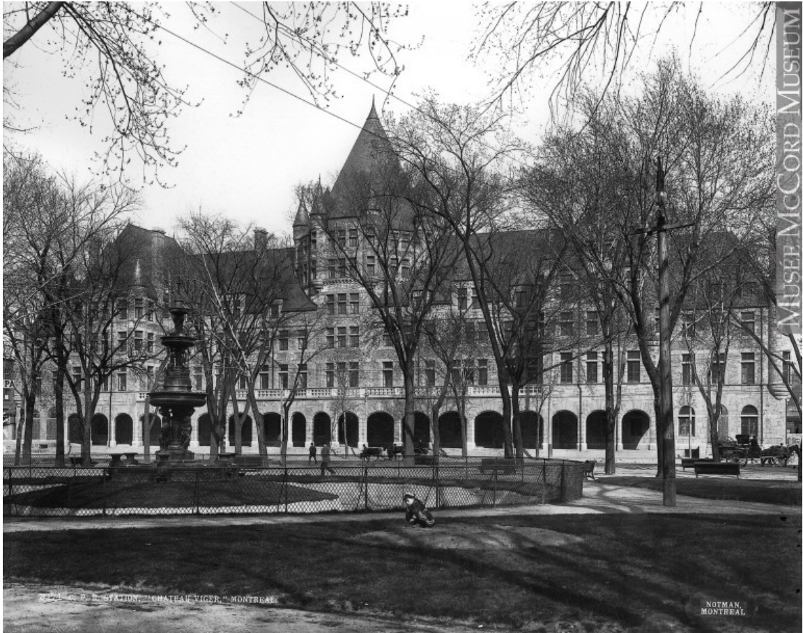
Place Viger railway station and hotel William Notman & Son. About 1901. Photograph Source: McCord Museum, Montreal
