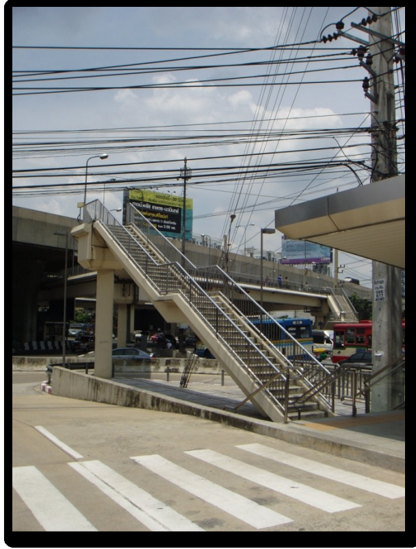
Figure 8: Lat Phrao Station Exit 4 pedestrian bridge
