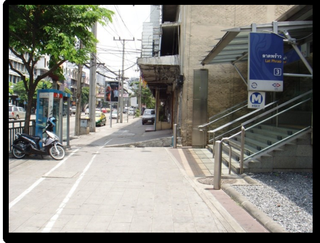
Figure 9: Lat Phrao Station Exit 3
