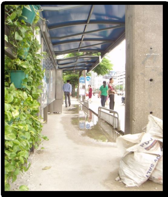
Figure 16: Bus Shelter at Lumphini Exit 2
