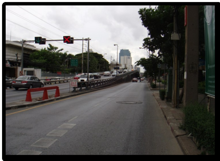
Figure 1: A Flyover bridge on Petchaburi road
