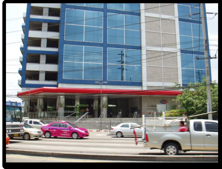
Figure 7: Lat Phrao Station Exit 4
