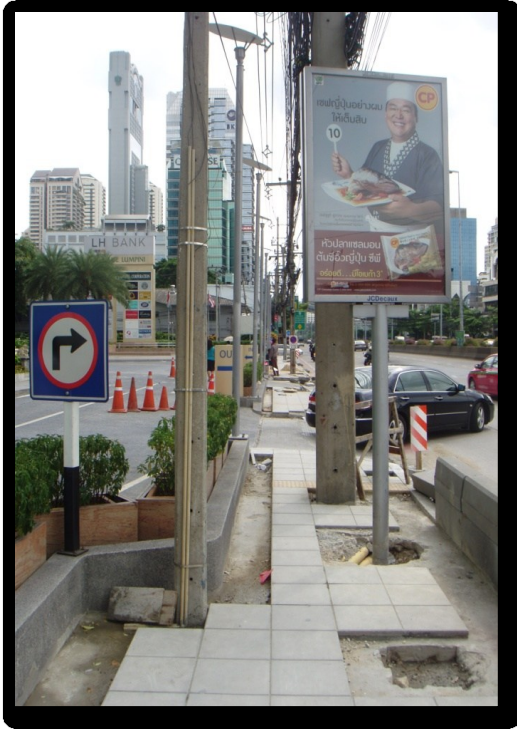
Figure 15: Obstructions and construction debris at Lumphini Exit 2
