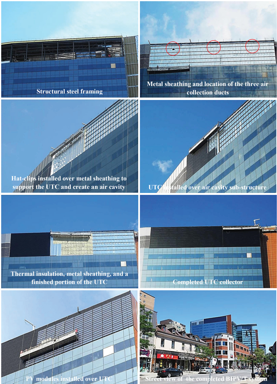
Figure 5.9: Construction sequence for the full-scale BIPV/T demonstration project.
