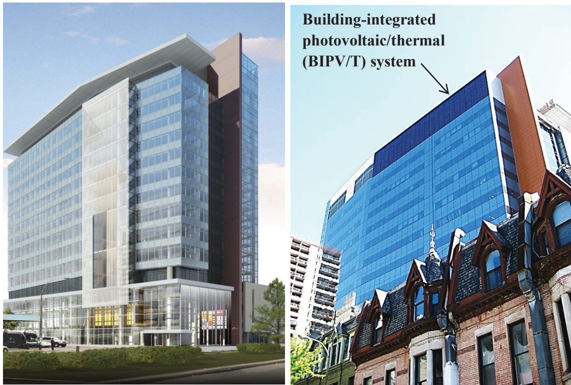
Figure 5.1: Conceptual drawing of Concordia University’s John Molson School of Business building (left). The full scale BIPV/T demonstration project installed on its near-south-facing façade (right).
