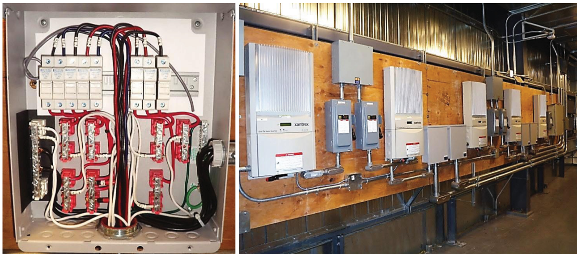
Figure 5.8: Wiring inside the combiner box (left). Xantrex inverter installation (right).
