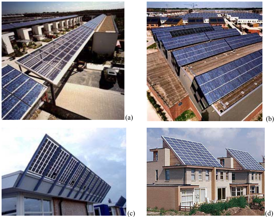
Figure 1.10, PV integration in Nieuwland, (a) on the roof of a parking lot; (b) in sport complex, (c) noise wall houses, (d) Prefab PV roofs (PV UPSCALE: Nieuwland, 2008).
