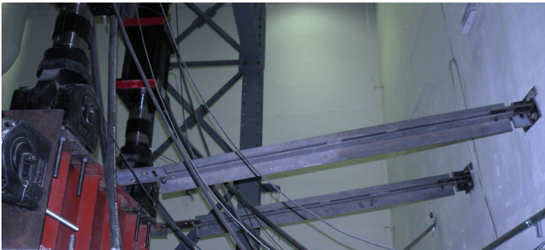
Figure 5.7 The steel braces to restrain the out-of-plane movement of the wall.
