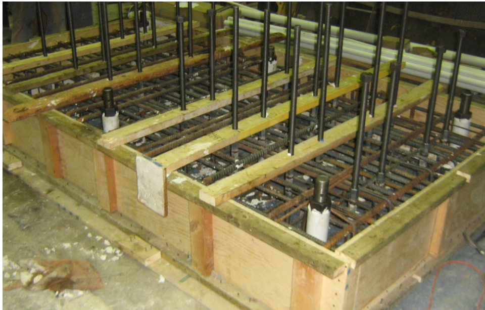
Figure 5.4 The rigid footing prior to the pouring of concrete.
