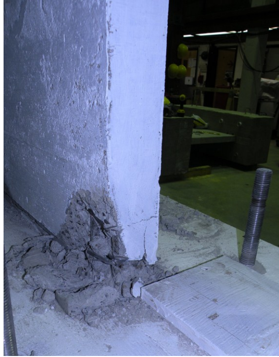
Figure 6.4 Concrete toe crushing of the CW.
