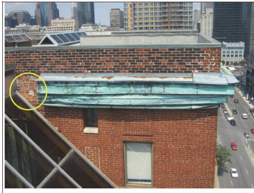
Photo No. 8 – Flashing at top of 12 th floor windows requires repair and localised spalled brick.
