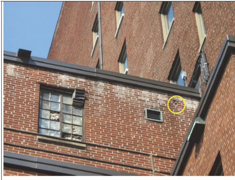
Photo No. 6 – Broken window panes and penetration hole on west elevation of roof Basin No. 6.
