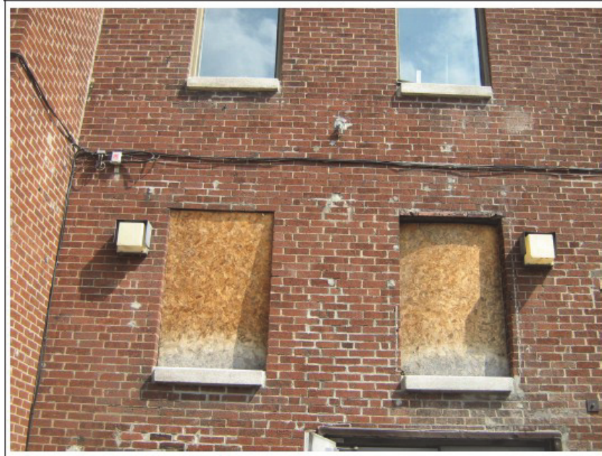
Photo No. 10 – Window openings located on the second floor of the north-western elevation currently enclosed with OSB (Oriented Strand Board) and re-pointing repairs.
