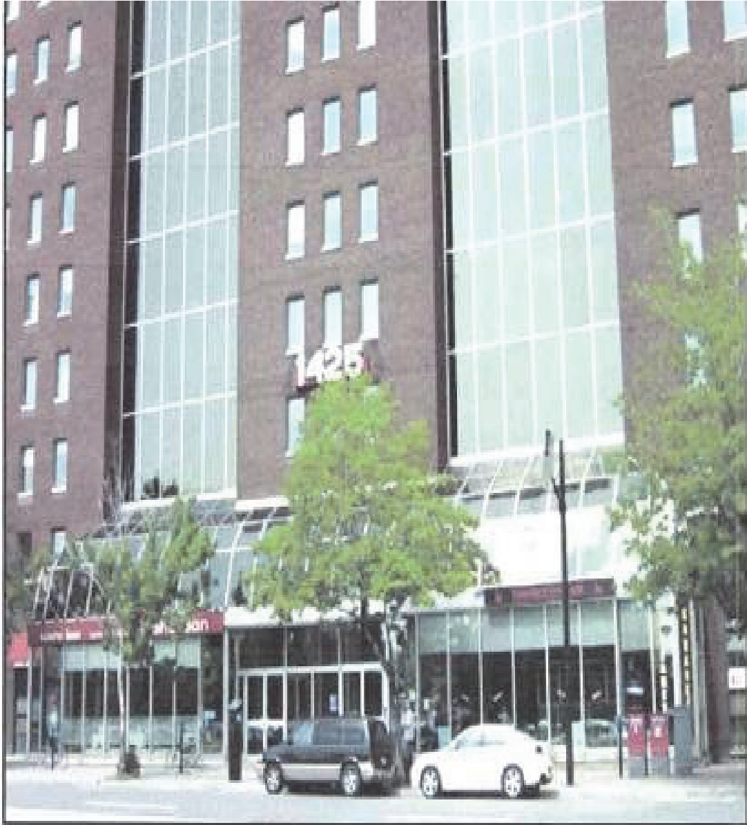
Figure 7-5 Building Photograph of 1425 Rene-Leveque Boulevard West, Montreal, Québec [Appendix C].
