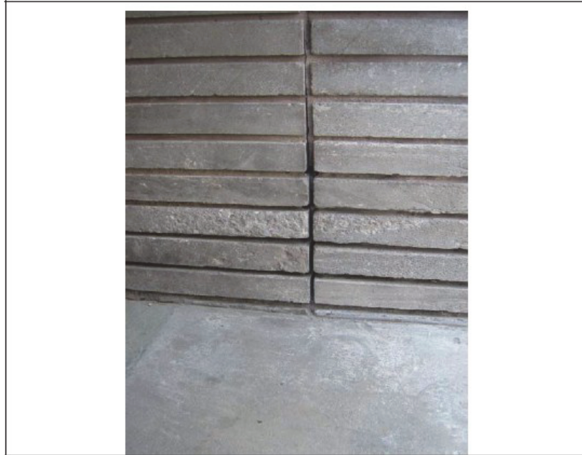
Photo No. 7 – Re-pointing work required to joints at the entrance of 1160 Bishop.
