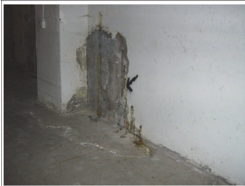
Photo No. 5 – Previous crack injection repairs to the foundation walls in the north-western basement.
