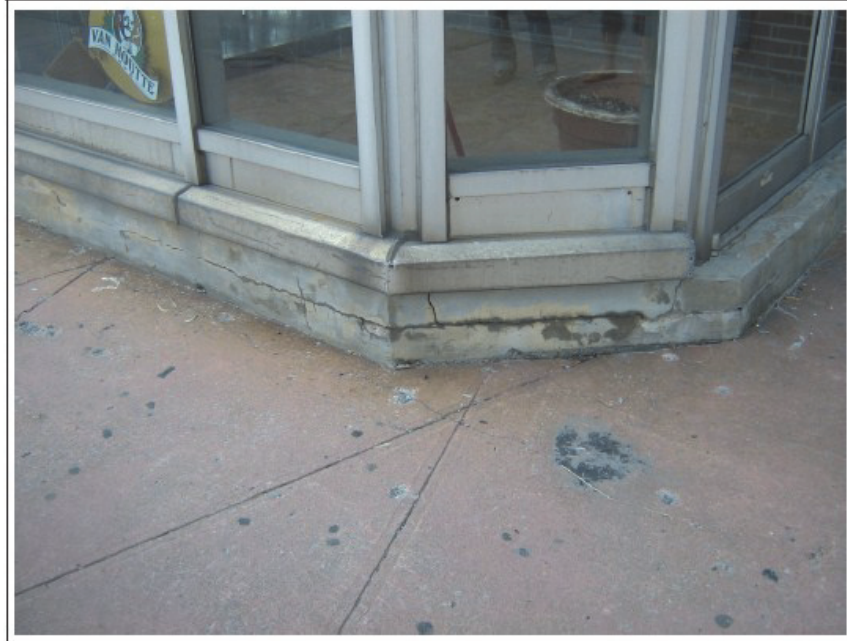
Photo No. 2 – Cracks to foundation wall located on south-eastern corner of the building.
