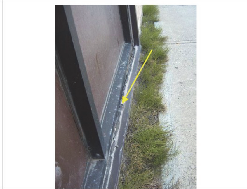
Photo No. 9 – deteriorated and pulled away caulking around window units on east elevation.
