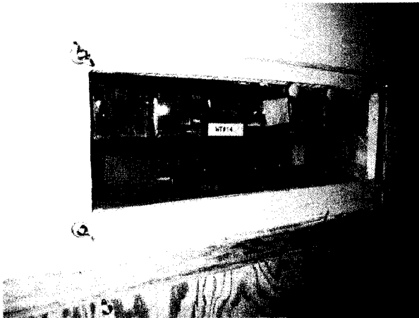
Figure 3-50. LC and water tray window installed
