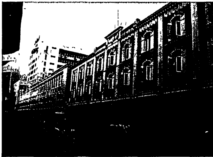
Figure 23 Traditional ‘Top-residential and Floor-commercial’ Building (Chen, Ming)
