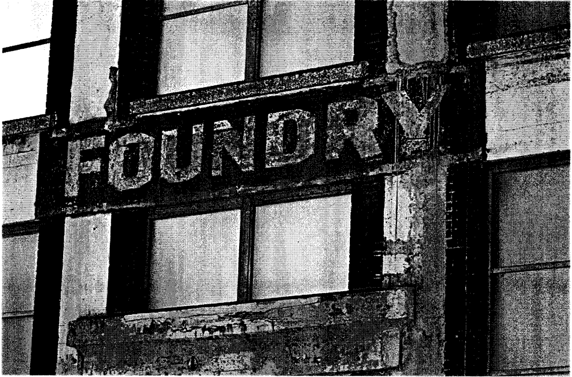
Fig. 11 Detail of exterior of Foundry after renovation. Source: photo taken by author, 2008.
