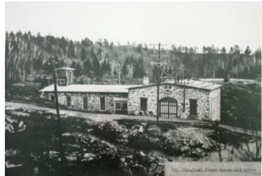
1.3.2 + 1.3.3 Old photographs show the first hydro-electrical power station, which was removed in 1950, leaving only the annex from 1904 (photo top: Anja Borck, bottom: Fonds Shawinigan Water and Power Company).
