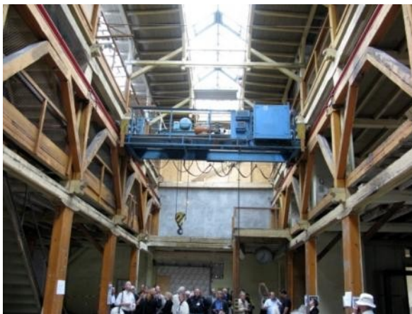
2.4.3 Wood construction of the knitting machine factory in Kappel, Saxony (photo: Anja Borck).
