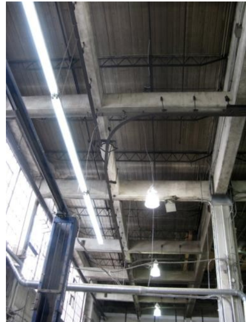
3.6.1.6 + 3.6.1.7 Interior front part with concrete frame (left) and interior back part (top) with steel frame and overhead rails (photos: Anja Borck).
