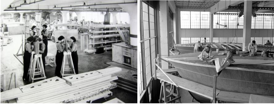
3.6.1.3 + 3.6.1.4 Women fitting boards at the CPBC (left), workers covering the hulls of motor torpedo boats under construction with linen fabric (right), (photo left: curtsey of Bernard Goldberg, right: Library and Archives Canada, MIKAN no. 3205298).
