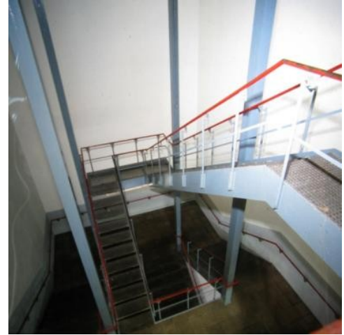
4.7.11+ 4.7.12 Interior, the ground floor structure is a reinforced concrete frame with low ceiling and short spans between the pillars. The stairs hang on four slender steel pillars. Photos were taken in 1996, after operations ceased (photo: Archives Regierungspräsidium Freiburg, Referat Denkmalpflege).
