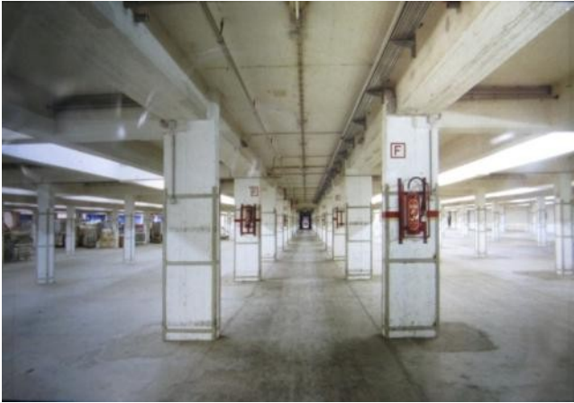
4.7.11+ 4.7.12 Interior, the ground floor structure is a reinforced concrete frame with low ceiling and short spans between the pillars. The stairs hang on four slender steel pillars. Photos were taken in 1996, after operations ceased (photo: Archives Regierungspräsidium Freiburg, Referat Denkmalpflege).
