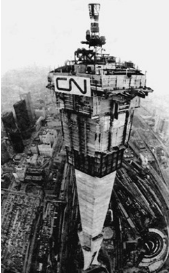
1.5.8 The slipform construction, which engineers developed to build grain elevators, was used for Toronto's CN Tower (1972-1976). The photo shows the tower under construction in 1974 with the mould visible which is moved upwards during the construction process (photo: unknown).
