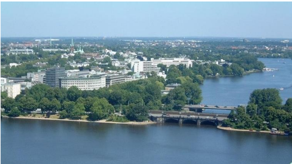
4.3.2 The Old Lombards Bridge (front) and the 1953 inaugurated New Lombards Bridge (behind), renamed Kennedy Bridge in 1963 (free span of 94 meters) cross Hamburg's Alster Lake. Bernhard Hermkes designed the Kennedy Bridge with engineer Hans Konrad Havemann (photo: Wolfgang Meinhart).
