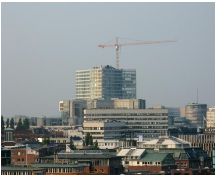
4.2.20 + 4.2.21 The Unilever Tower (Emporio Tower since 2012) during renovation and extension in 2009. The tower kept its heritage status after the modernization and two-floor extension (photo left: Anja Borck, right: HPP Architects).
