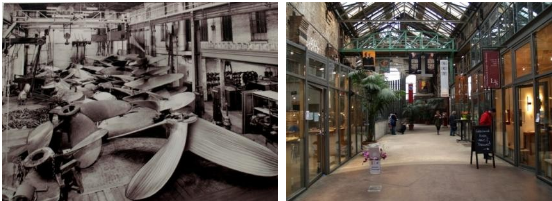
0.7 + 0.8 The ship propeller factory Zeise, once the largest in Germany, closed its doors in 1978 after hundred ten plus years in operation. It stood vacant for nearly twenty years before the architects of me di um architekten helped to redeveloped it into a multi functional commercial and office building. In the floor, the large pits for the molds remained visible, the walls still show traces of the building's age (photos: Kay's Weblog).
