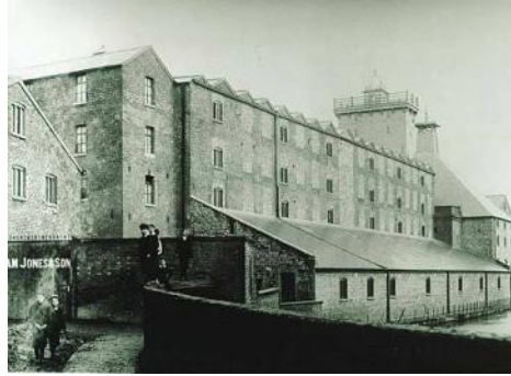
2.4.1 + 2.4.2 Ditherington Flax mill built in 1796, with the first known iron skeleton frame (photos: unknown).
