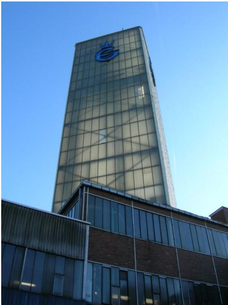
4.4.14 The translucent tower features the so-called Gerrix sign, a crowned “G”, once a common imprint on glass bottles in Germany (photo: Archives Untere Denkmalschutzbehörde Düsseldorf).
