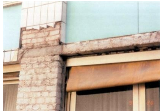
4.6.15 + 4.6.16 The high-rise administration building exchanged the old glass sheets with enamelled metal sheets. An extra layer of insulation pushed the windows deeper into the facade (photo left: Anja Borck, right: Archives Untere Denkmalbehörde Köln).
