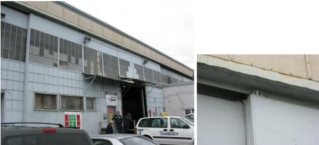
3.6.1.11 + 3.6.1.12 Sliding door were still in place in 2013 but blocked by later extensions (photo: Anja Borck).
