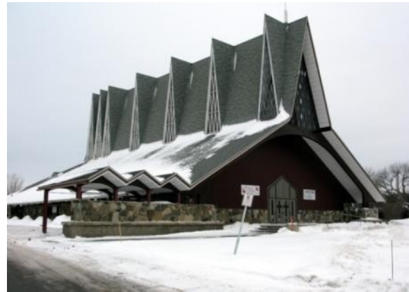
3.3.9 Saint Edward of Canterbury Church in Pointe-Claire's neighboring municipality, Beaconsfield, by Roger d'Astous was inventoried by 2013 but has not received legal heritage protection. Industrial sites, normally associated with a lower heritage priority, may need to wait long for recognition (photo: Anja Borck).
