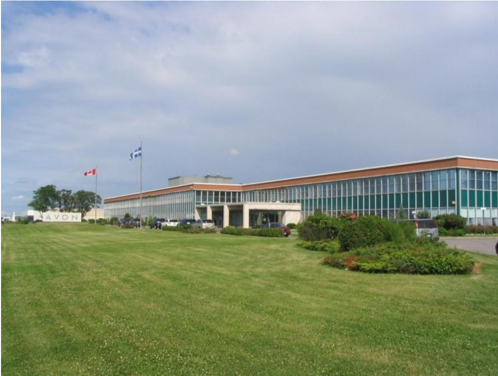
3.2.1 Avon Building in Pointe-Claire – of heritage interest since 2004 on a municipal level (photo: curtsey of Archives City of Pointe-Claire).
