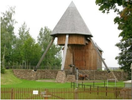
3.6.3.5 + 3.6.3.6 Reconstructed horse gin Rudolphschacht Lauta, near Marienberg, Saxony, used for the vertical transportation of loads inside the mine shaft. They were once a common feature at farms and in mining industries, in Germany all but one disappeared (photos: Anja Borck).
