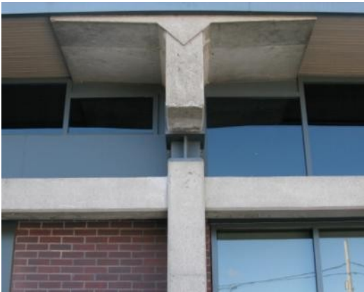
3.3.8 Detail of steel brackets for concrete beams at the Norman Wade building, emphasizing the frame construction (photo: Anja Borck).
