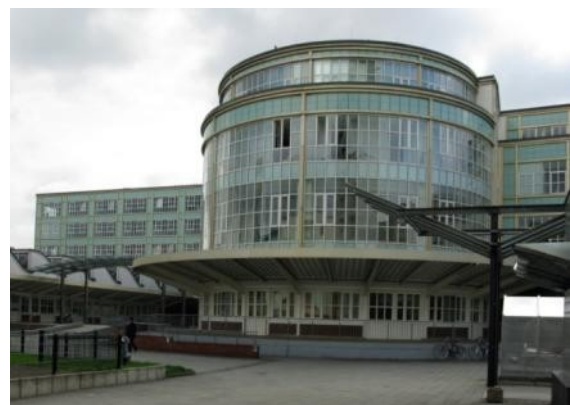
4.6.11 + 4.6.12 The warehouse before renovation and afterwards. Today, bright white window frames on the ground floor and a row of opaque glass to hide the concrete floor slab add visual weight to the building (photo left: Archives Untere Denkmalbehörde Köln, right: Anja Borck).
