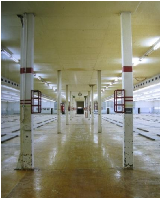
4.7.11+ 4.7.12 Interior, the ground floor structure is a reinforced concrete frame with low ceiling and short spans between the pillars. The stairs hang on four slender steel pillars. Photos were taken in 1996, after operations ceased (photo: Archives Regierungspräsidium Freiburg, Referat Denkmalpflege).
