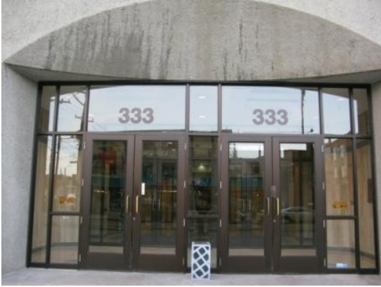
3.6.5.7 + 3.6.5.8 Entrance and foyer of 333 Chabanel Street West with terrazzo floors and travertine siding on the walls (photos: Anja Borck).
