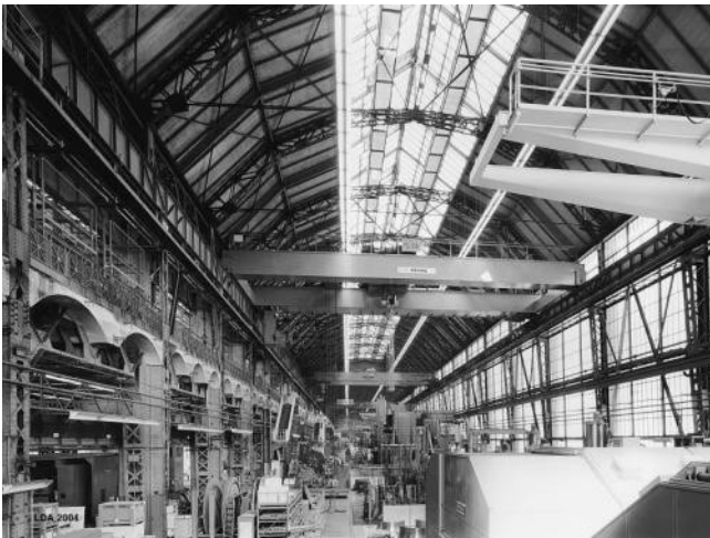
2.6.9 + 2.6.10 AEG Turbinen Hall in Berlin Morbit from 1909 by Peter Behrens, exterior and interior, used as storage when the photo was taken in 2004 (photo top: LDA, bottom: LDA).
