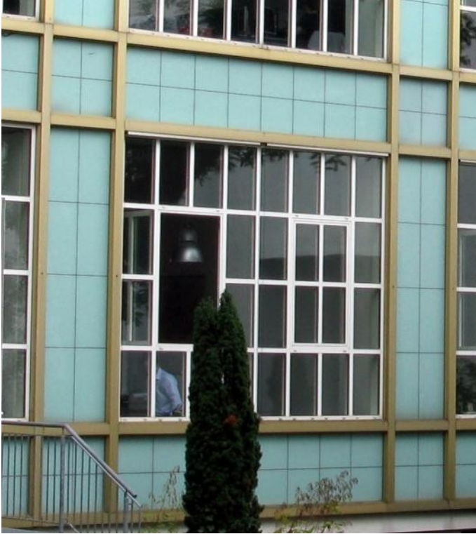
4.6.13 + 4.6.14 New turquoise safety glass sheets replace the glass tiles. Where larger areas of tiles had been mounted without a frame, new fixtures support the larger glass-sheets (photos: Anja Borck).
