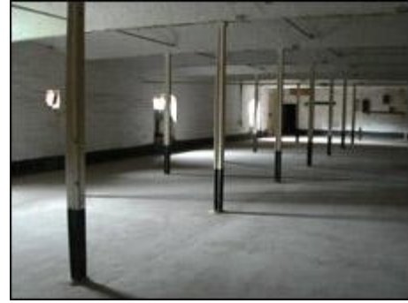
2.4.1 + 2.4.2 Ditherington Flax mill built in 1796, with the first known iron skeleton frame (photos: unknown).
