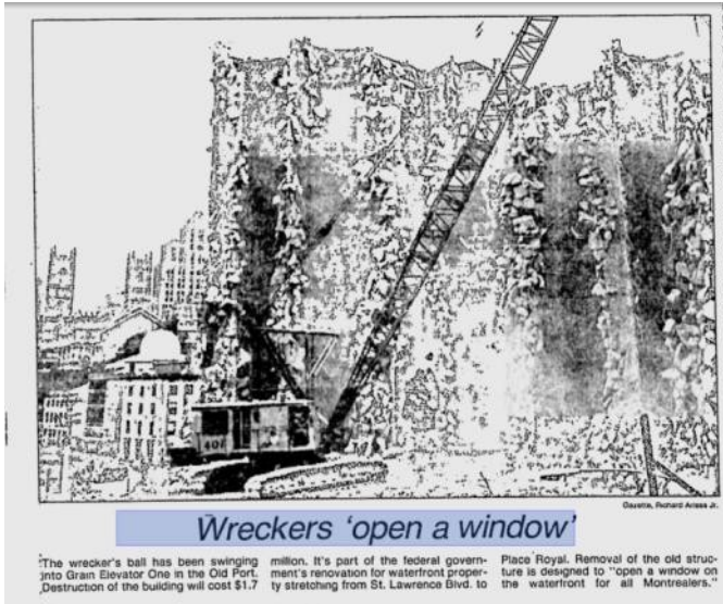
1.5.11 The Montreal Gazette reported on Thursday August 18, 1983 on the demolition of the Grain Elevator No 1.
