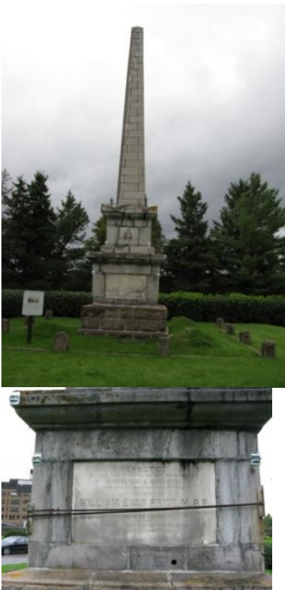
1.6.8 The Price Monument from 1882 in Chicoutimi showed clear signs of deterioration in spring 2011 (photos: Anja Borck).
