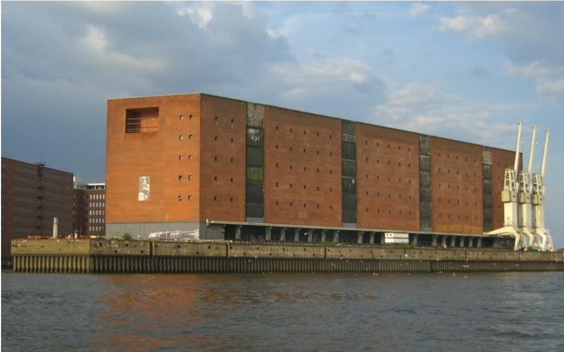
4.2.1 Kaispeicher A in the harbor of Hamburg seen from the Elbe River in c. 2000 (photo: unknown).
