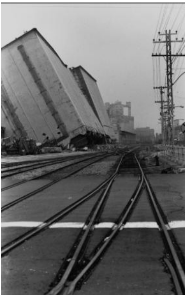
1.5.9 + 1.5.10 The failed demolition of the Grain Elevator No 2 in 1978. After a second, successful attempt, only some foundation work (arrow) remained visible, which grass had covered by 2012 (photo left: unknown, photo right: Société du Vieux-Port de Montréal).
