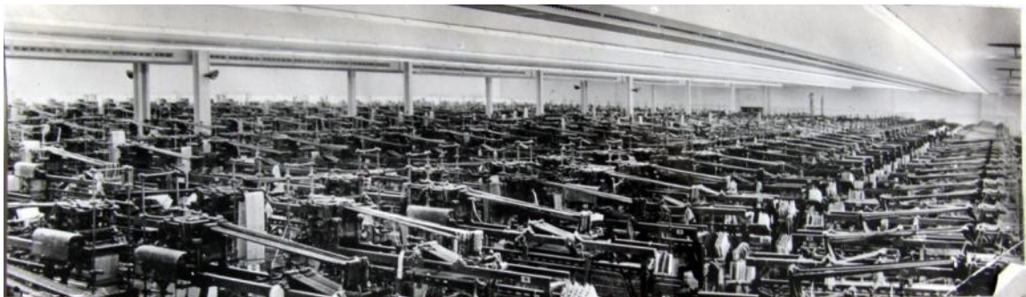
4.7.10 When the company opened in 1950, they produced fashionable handkerchiefs with more than five hundred looms. At the beginning of the 1960's, the size of the production hall doubled (photo: Ibs Ingenieurbüro für Bauwesen Schweizer).
