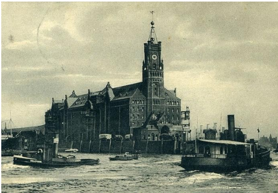
4.2.6 + 4.2.7 The old Kaispeicher A, photo around 1910, with the widely visible time signal: A ball, one meter in diameter, would fall three meters at noon, Greenwich time, exact to a tenth of a second. Ships could adjust their navigation instruments to it (photo: unknown, drawing: Schramm).
