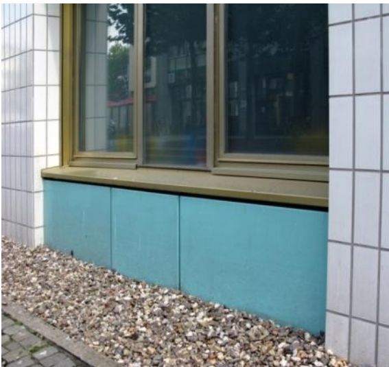
4.6.15 + 4.6.16 The high-rise administration building exchanged the old glass sheets with enamelled metal sheets. An extra layer of insulation pushed the windows deeper into the facade (photo left: Anja Borck, right: Archives Untere Denkmalbehörde Köln).
