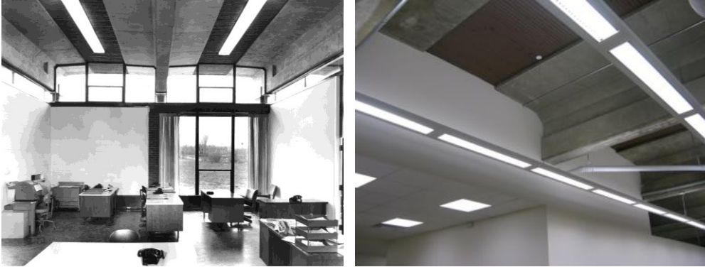
3.3.6 + 3.3.7 Interior of the Norman Wade building as in 1961 (left) and how it was changed during the renovations in 2012, disrupting the formerly visible main beam (right), (photo left: Archives Le Groupe Arcop, right: Anja Borck).
