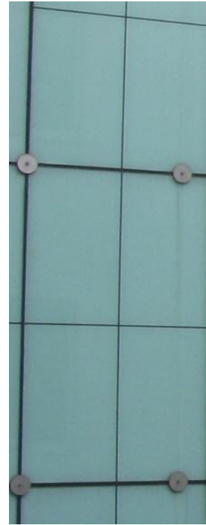
4.6.13 + 4.6.14 New turquoise safety glass sheets replace the glass tiles. Where larger areas of tiles had been mounted without a frame, new fixtures support the larger glass-sheets (photos: Anja Borck).
