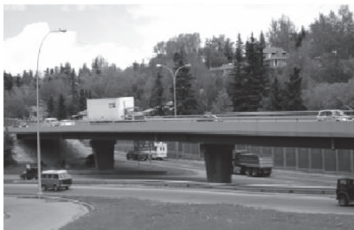
Figure 4.2 Overall View of Crowchild Trail Bridge, Calgary, Alberta (VanZowl et al. 2008)
