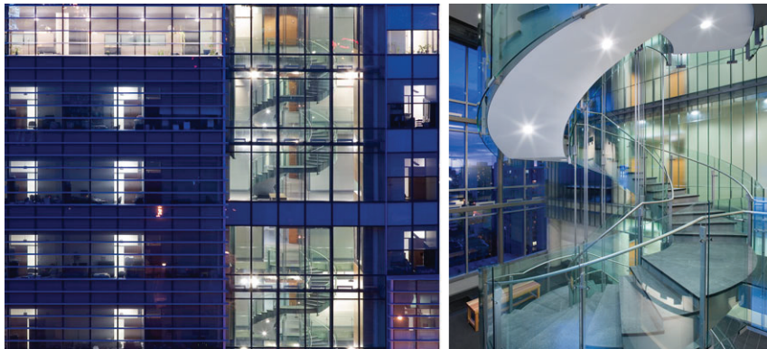
Fig. 7: EV Building, Guy Street facade at dusk (left), spiral stairwell (right); photo credit: Tom Arban; retrieved from http://www.kpmb.com .
