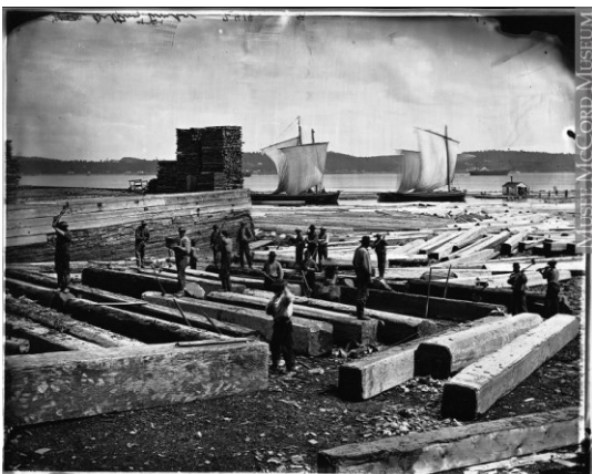
Fig. 4.6 , Butting square timber, Quebec City, QC, 1872 . William Notman (1826-1891), I-76312. McCord Museum, Montreal.
