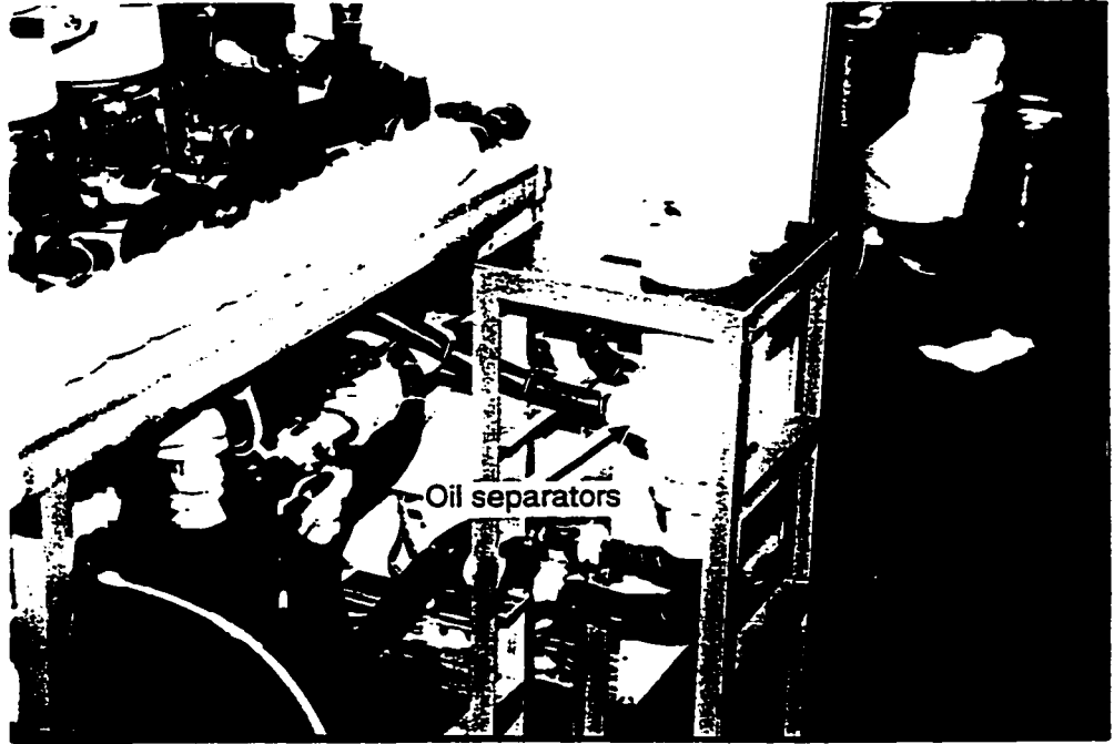
Figure 2.5 Oil separators
