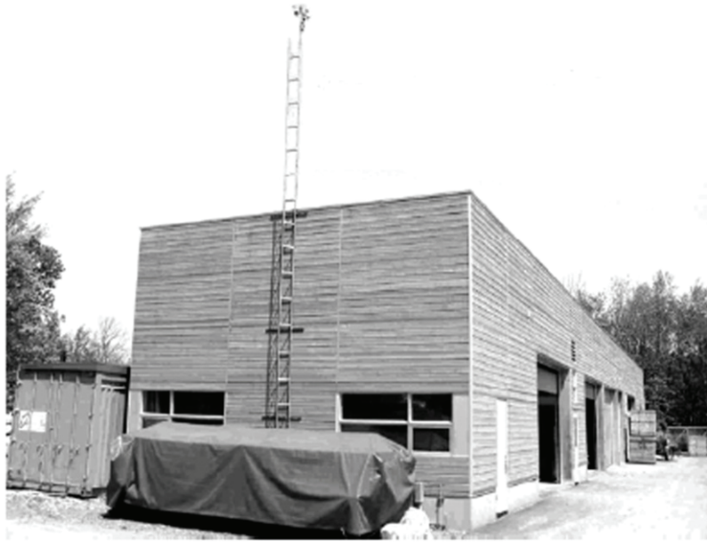
Figure 2.8 Experimental structure located in Saint Foy, QC (after Doudak et al. 2005).
