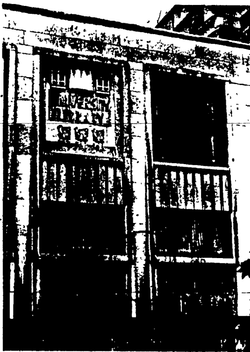
FIG. 3.33: Type 1.3, typical weathering pattern likely to occur around projecting frames.
