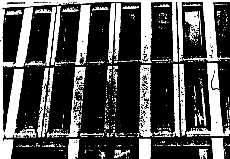
FIG. 3.49: Type 1.4.2, examples of vertical sectional profile that interrupt water flow from one storey to another.
