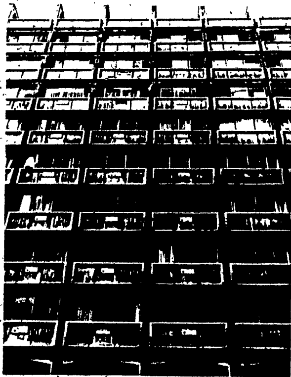
FIG. 3.23: Wetting by driving-rain, and hence washing action, is limited to the top storey of this facade.
