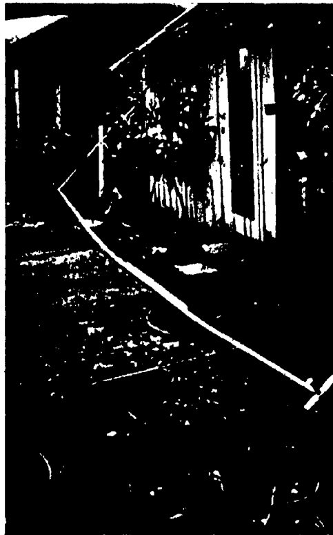
Fig. 3.13 - Self-Helper Copying the Perimeter of the House Using the Aluminium Frame
