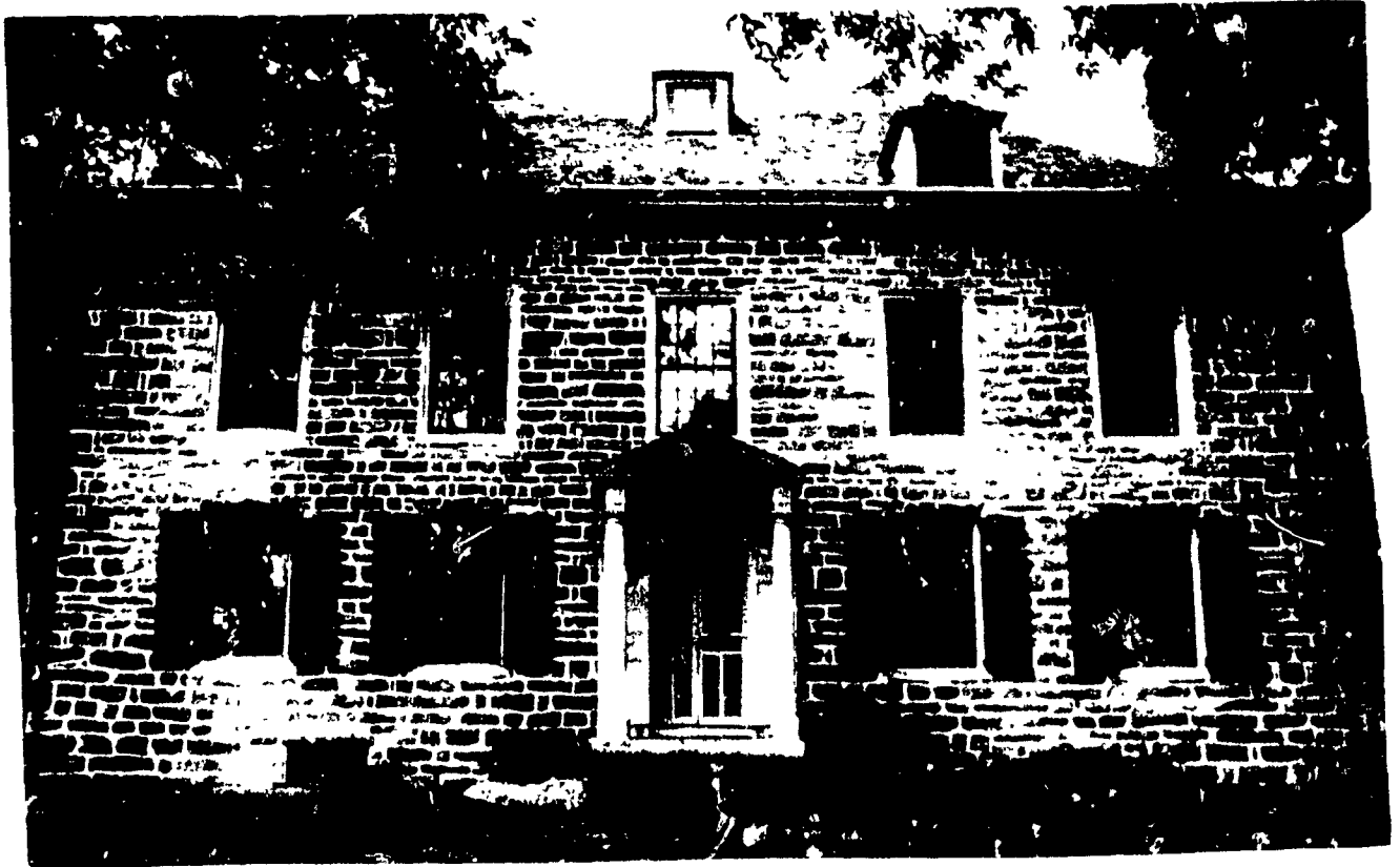
Figure 5. Fort Johnson Entrance Front
