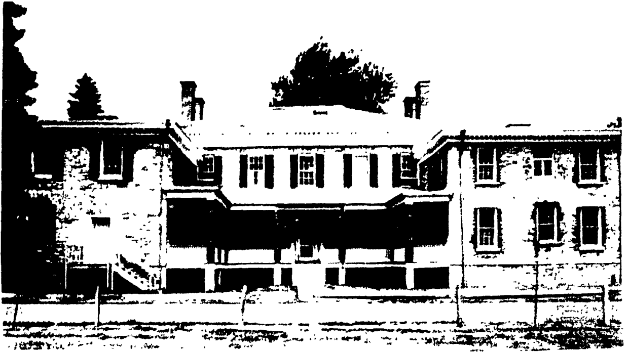
Figure 15. Guy Park River Front
