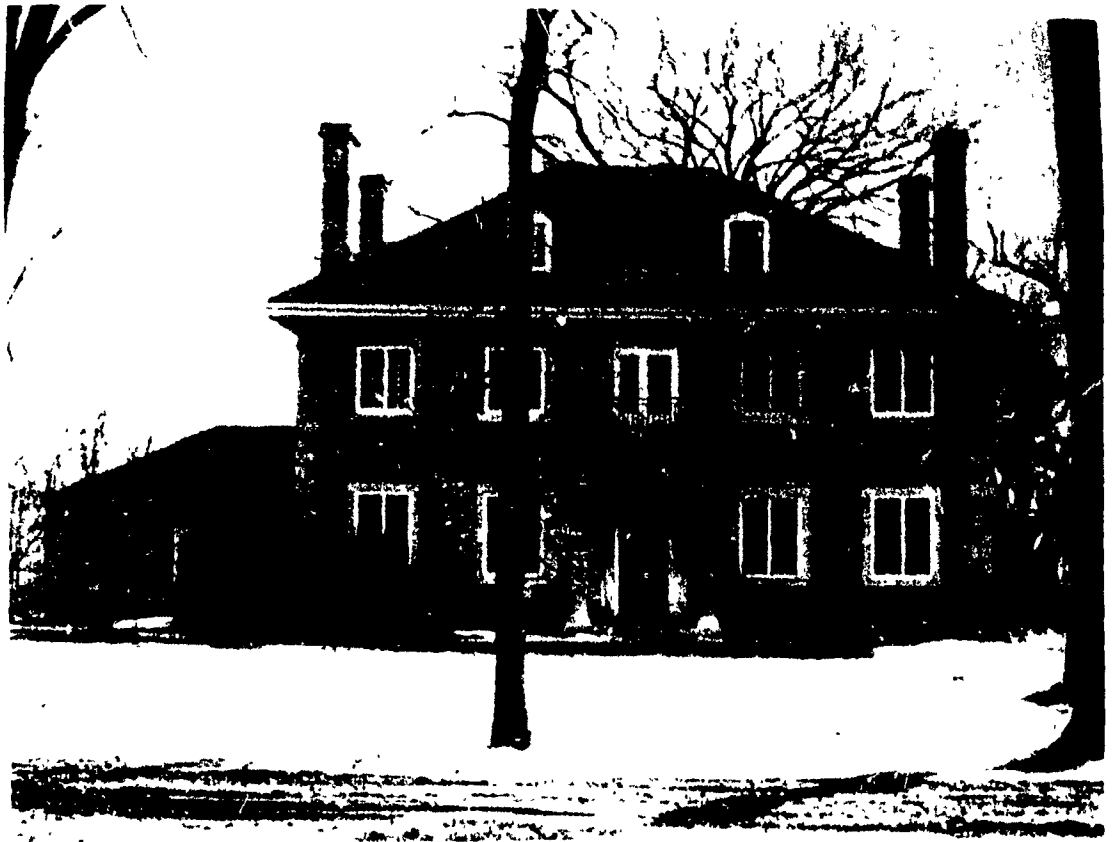
Figure 28. The Johnson Manor House, St. Mathias, PQ, Entrance Facade
