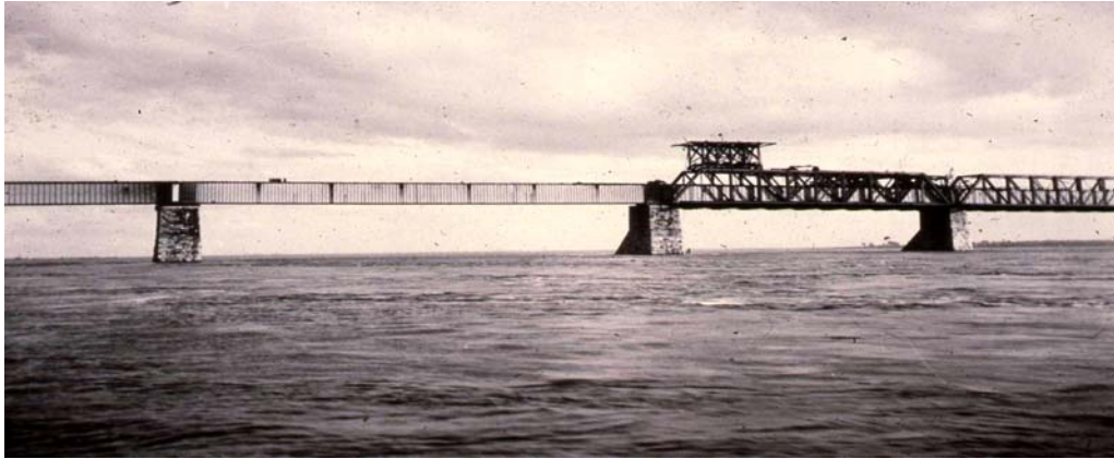
Figure 3. Substitution on the 2 km (25span) Victoria bridge in 1898 of the steel truss spans (right spans) around the 1858 single-track tube (WI box-girder, left spans) was supported by a wider, higher construction frame (second span from right) directly resting on the piers; however, it could be rolled forward span by span, being supported on the tube [6] (Notman Photograph, McCord Museum, Montreal).
