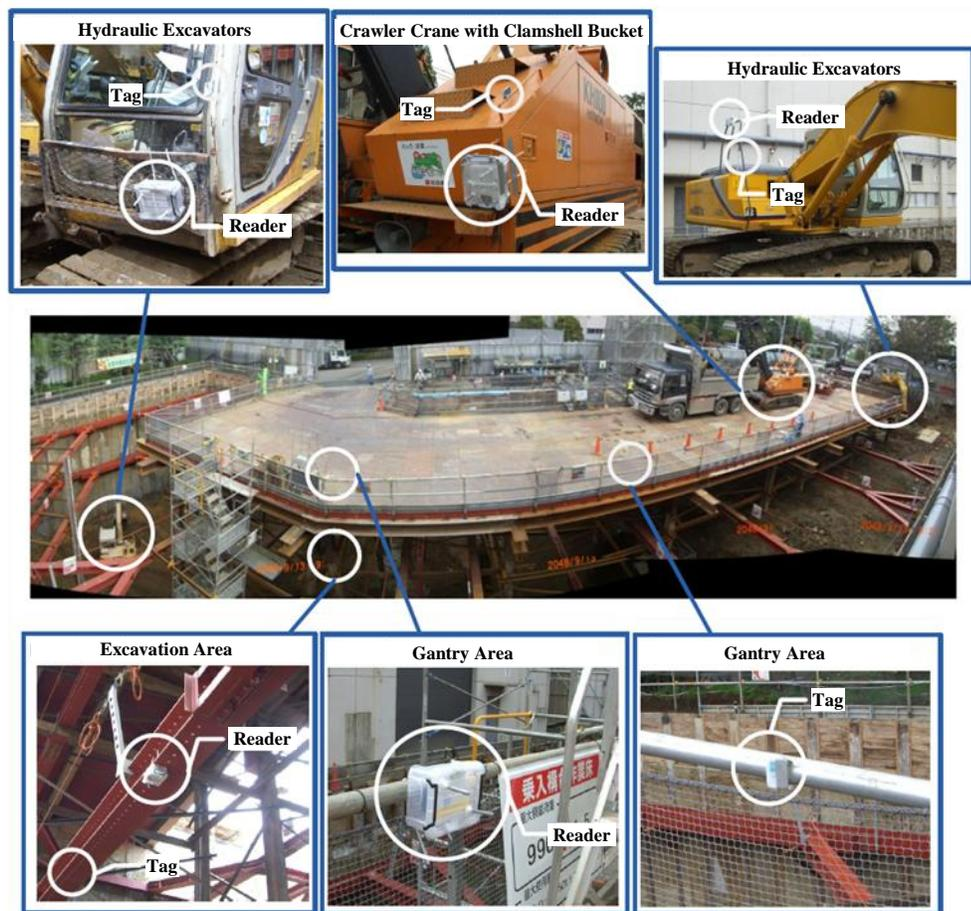
**Figure 2-19: Construction site equipped with RFID devices (Chae and Yoshida, 2008)**
