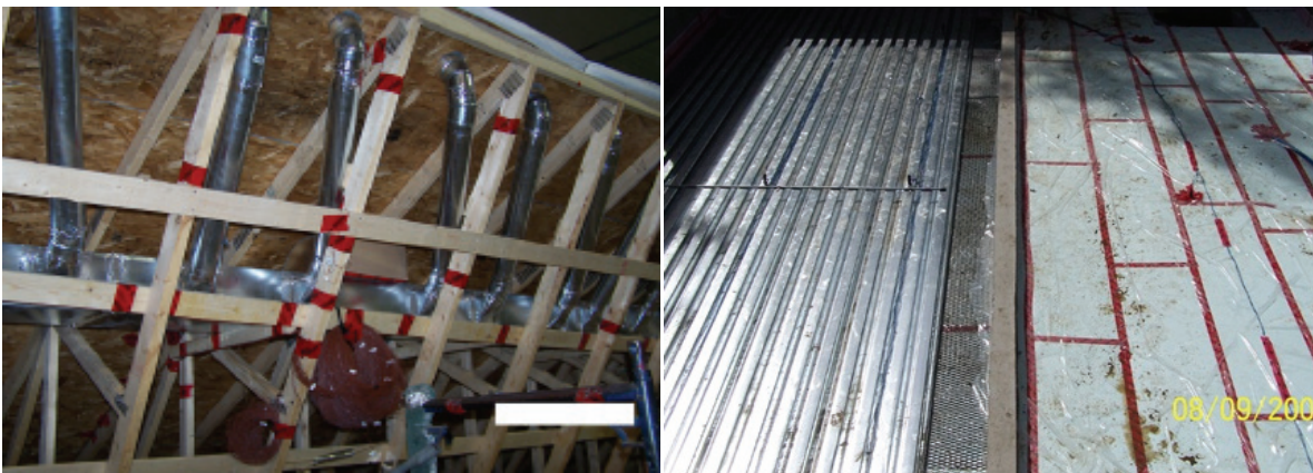
Figure 14-1: Photographs of the underside of the BIPV/T roof (left) and the ventilated slab before the concrete is poured on the decking (right)
