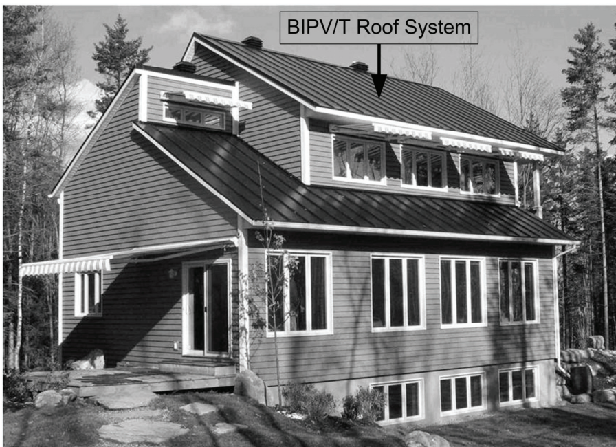
Figure 8-1: A photograph of ÉcoTerra house as seen from the south-west
