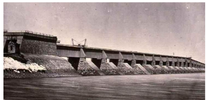
Fig. 2. Victoria Tubular Bridge, viewed from the northwest, showing the gradual incline towards the centre span and the piers for breaking ice floes. The thick protective abutment walls were removed when reconstructed in 1898 (Notman photograph, McCord Museum, Montreal; Triggs et al., 1992).
