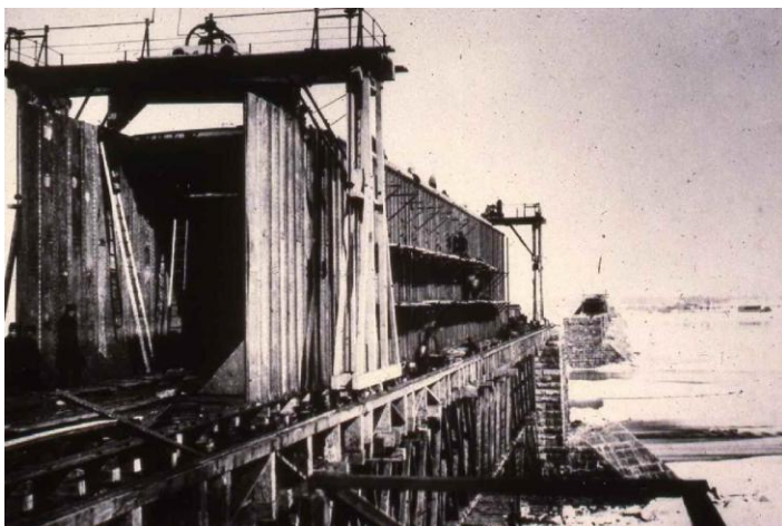
Fig. 9. Construction of the tubular (box-girder) centre span with a travelling gantry crane on a temporary timber truss over winter ice, as captured in a Notman photograph with the South Shore in the distance (McCord Museum, Montreal; Triggs et al., 1992).
