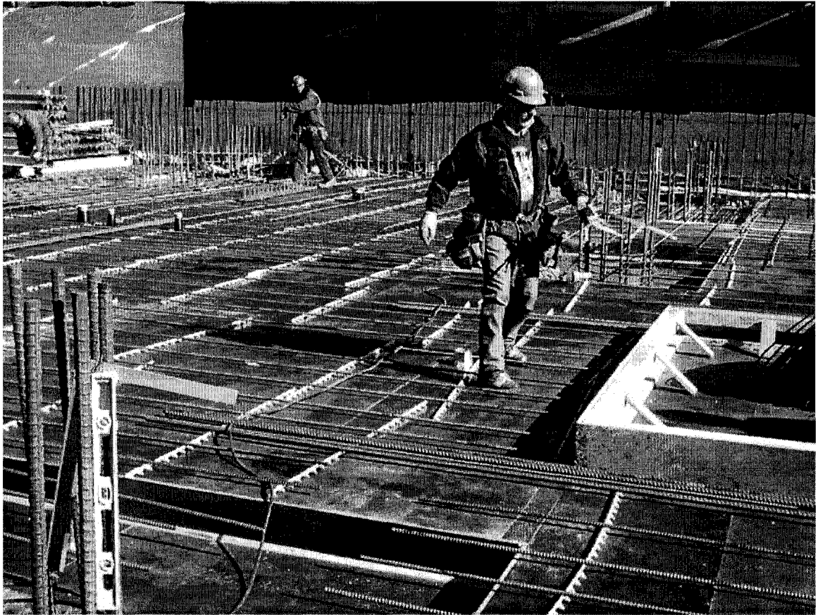
Figure 3.39 Reinforcing bars for slab (Concordia SGW site)
