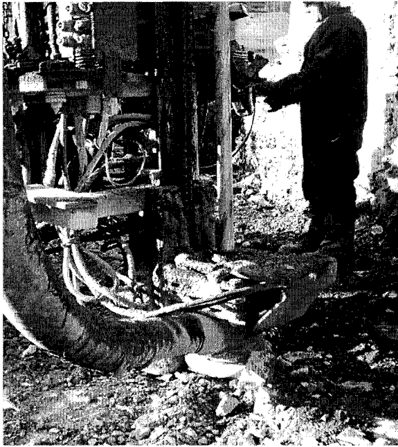
Figure 3.22 Locating aiguilles
