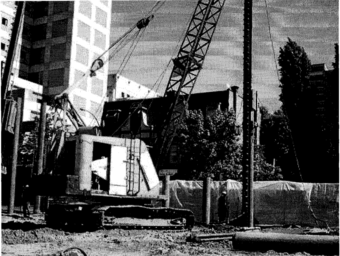
Figure 3.7 Link-Belt LS-98 pile driver
