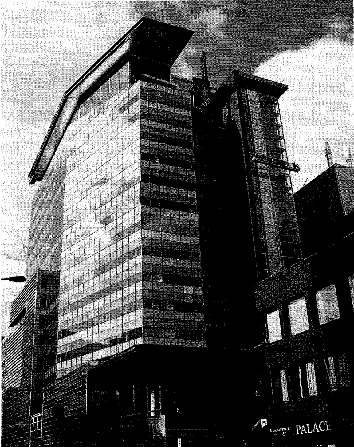
Figure 3.2 Engineering, Computer Science and Visual Arts Complex
