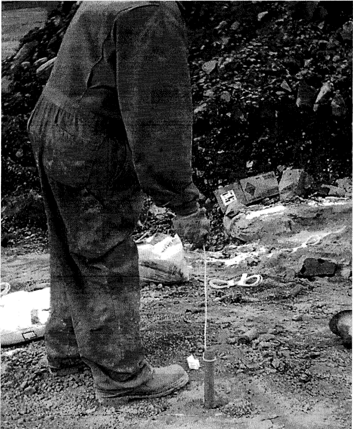
Figure 3.26 Placing cap and Powerditch primer
