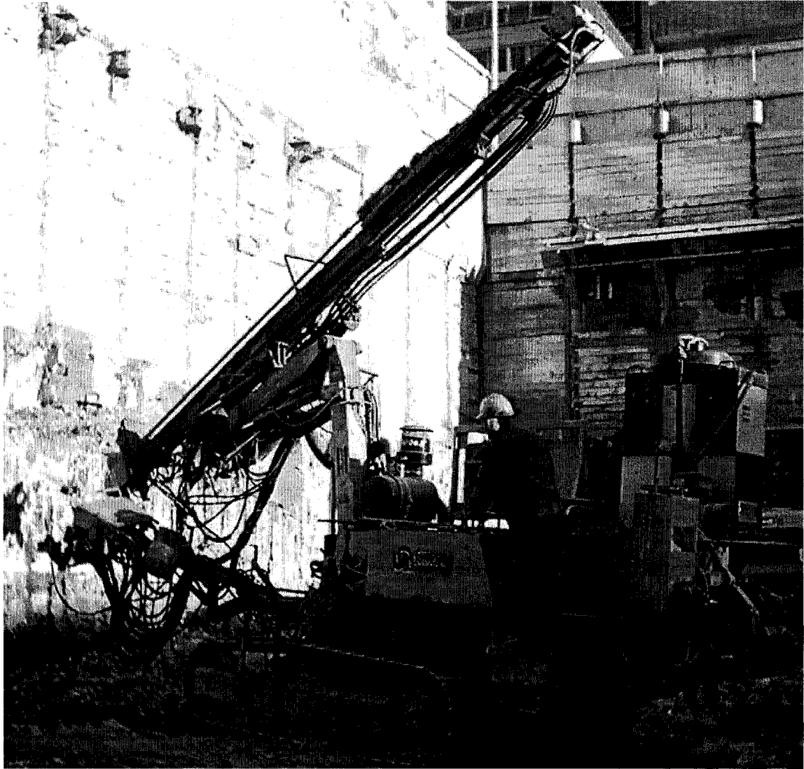
Figure 3.20 ROC 722HC-01 drilling machine
