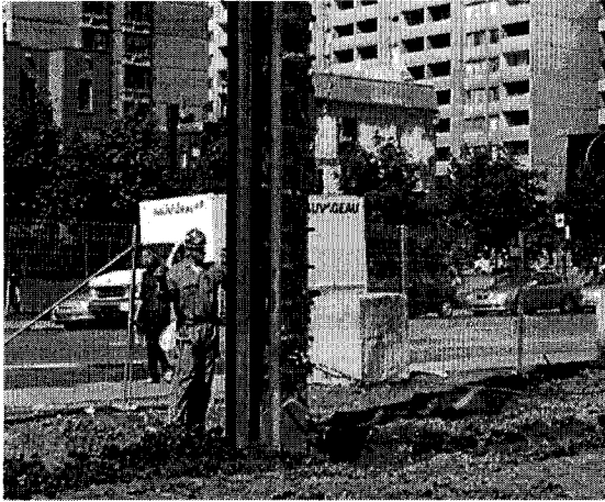
Figure 3.9 Checking verticality
