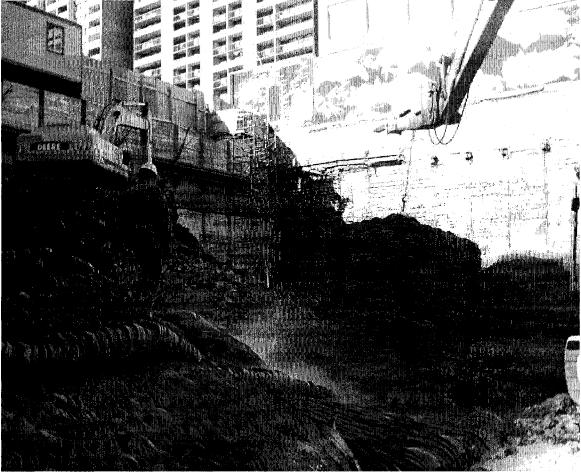
Figure 3.37 Removing mats after blasting
