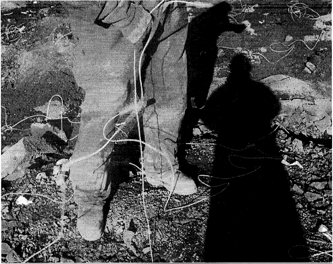
Figure 3.30 Connecting caps (25 ms delay each)
