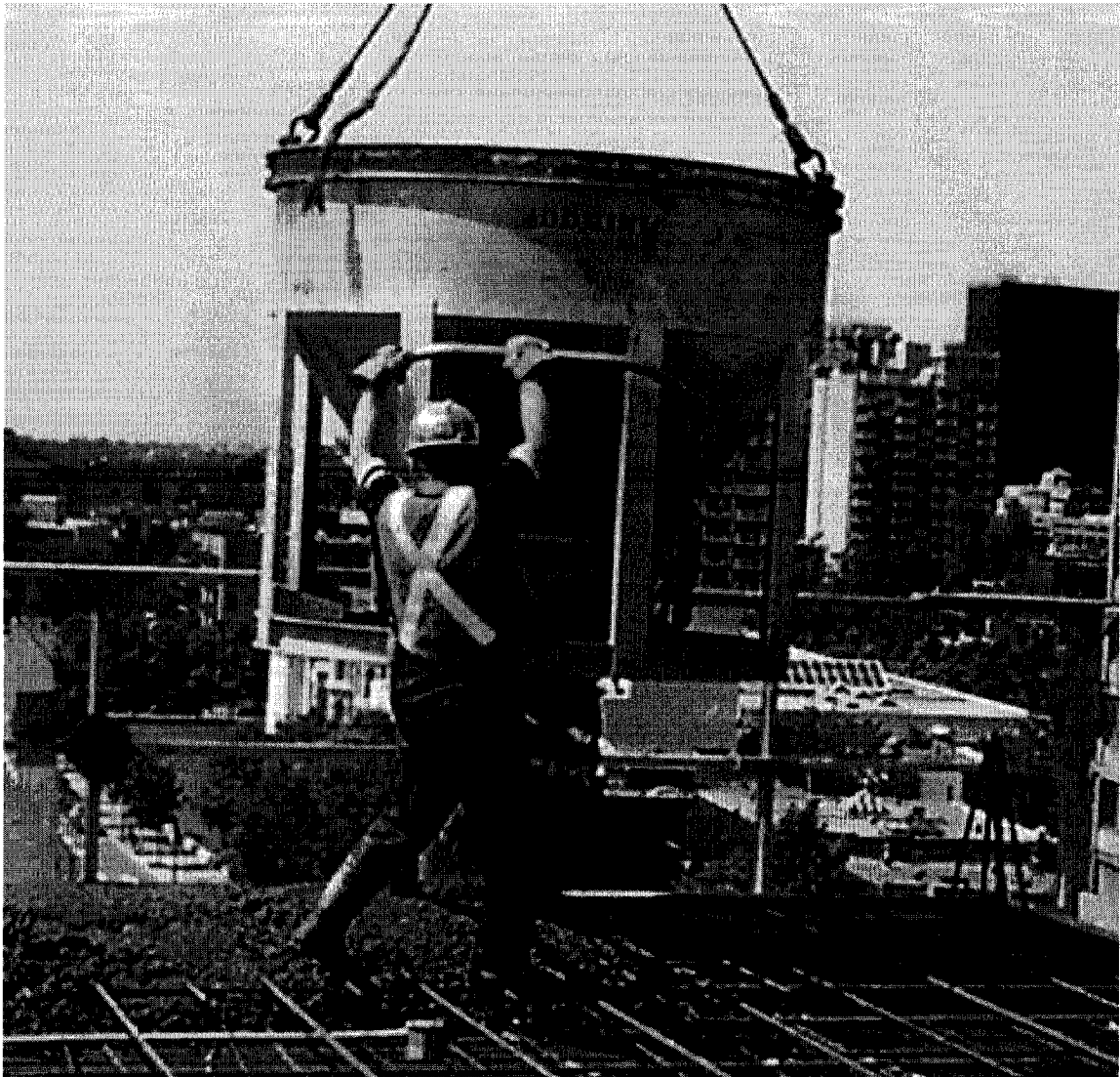
Figure 3.45 Pouring concrete by bucket
