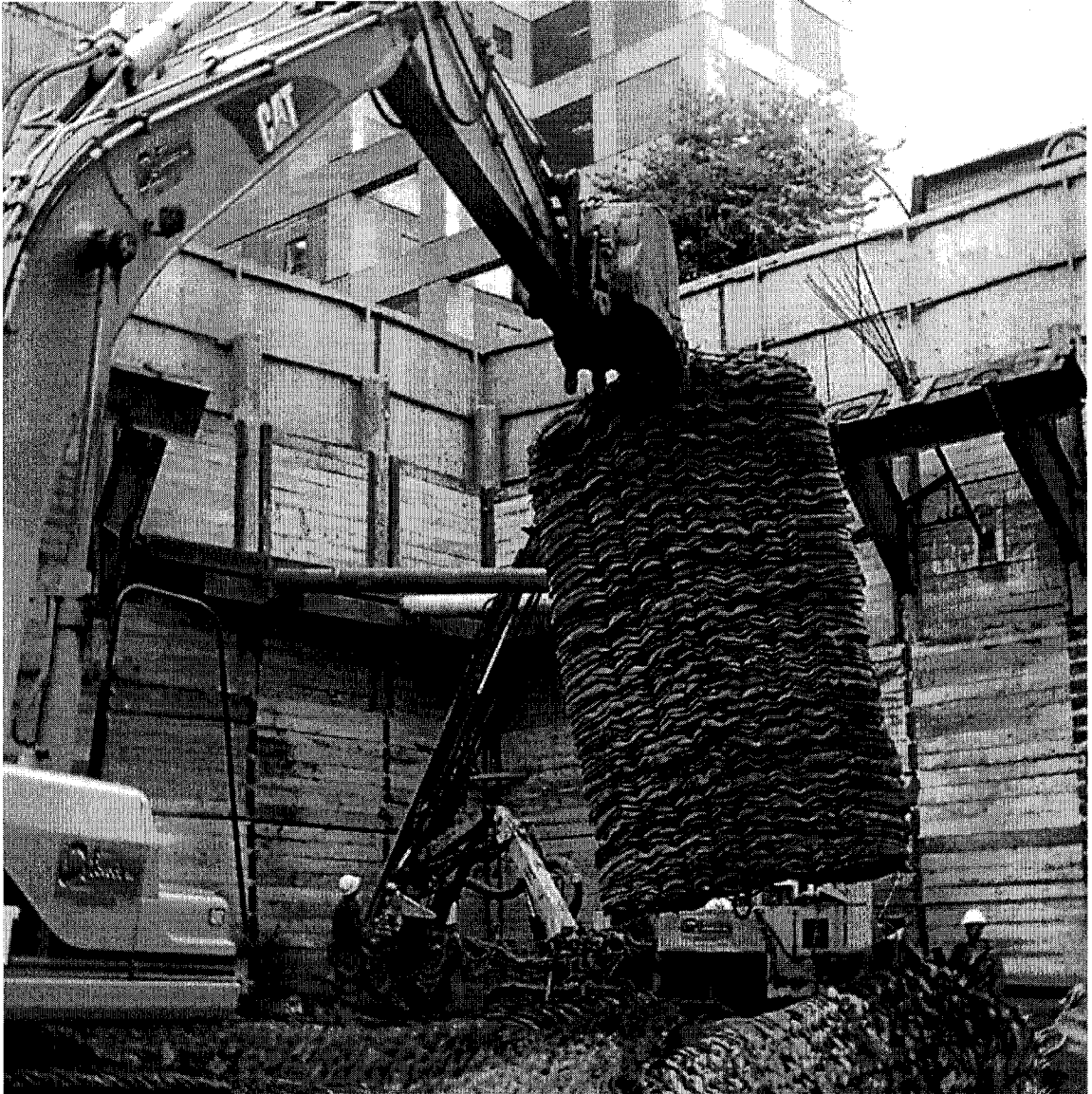
Figure 3.36 Placing rubber mat
