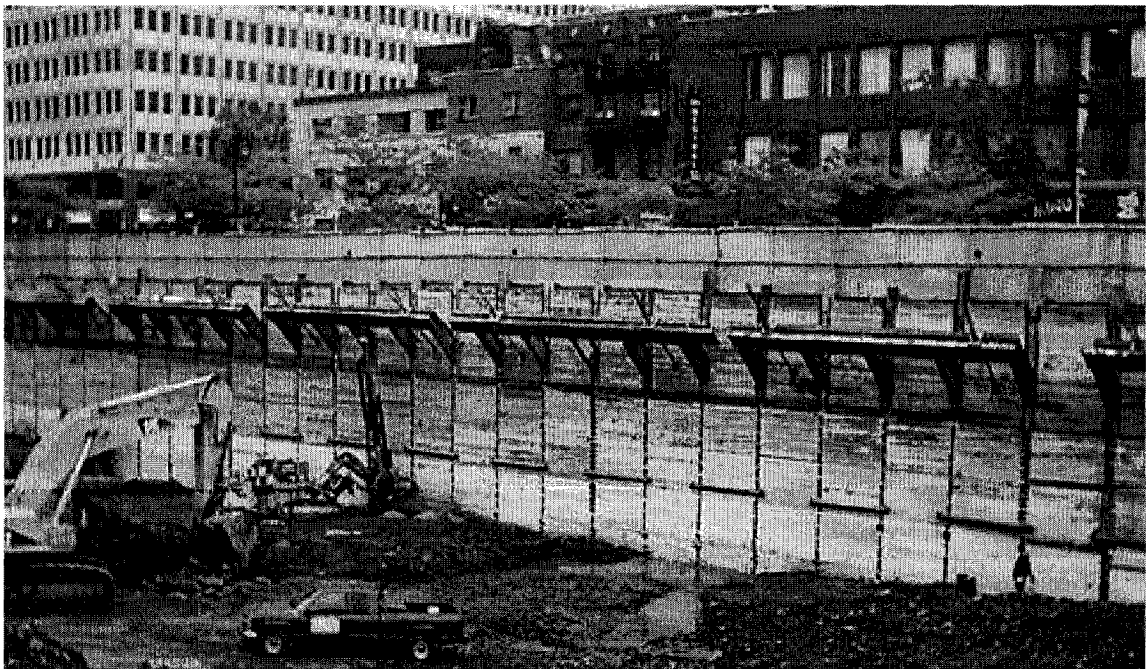
Figure 3.38 Completed shoring system in SGW site
