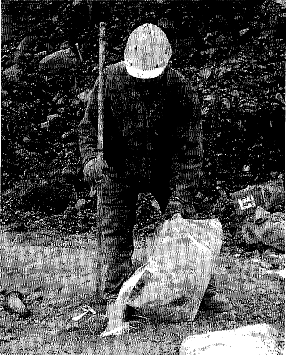
Figure 3.27 Placing dynamite and tamping
