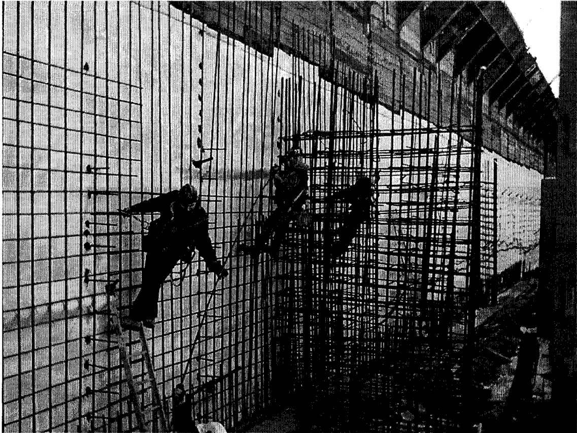
Figure 3.41 Reinforcing bars for wall (Concordia SGW site)
