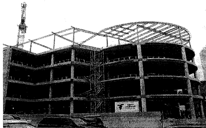
Figure 7.4 ETS building under construction
