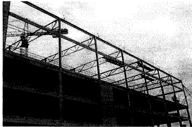
Figure 7.16 ETS building: actual Structural System under construction
