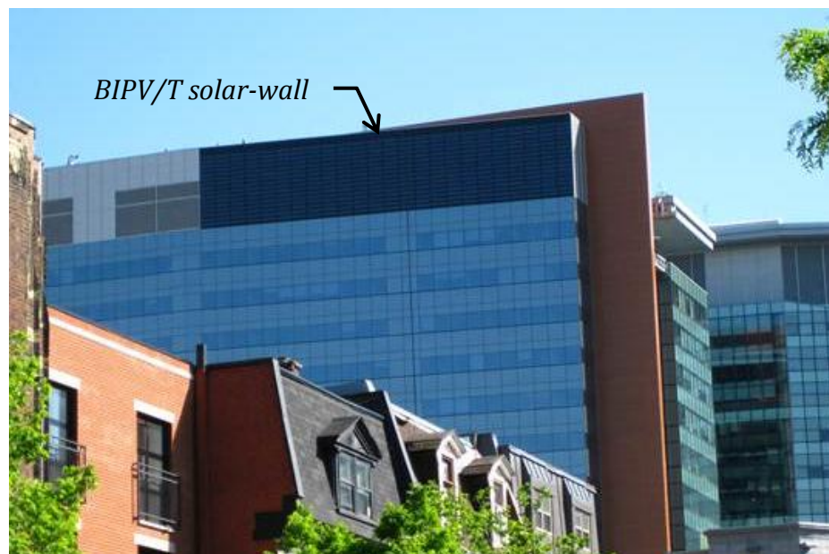
Figure 1.3: The John Molson School of Business building housing the building-integrated PV/thermal system
