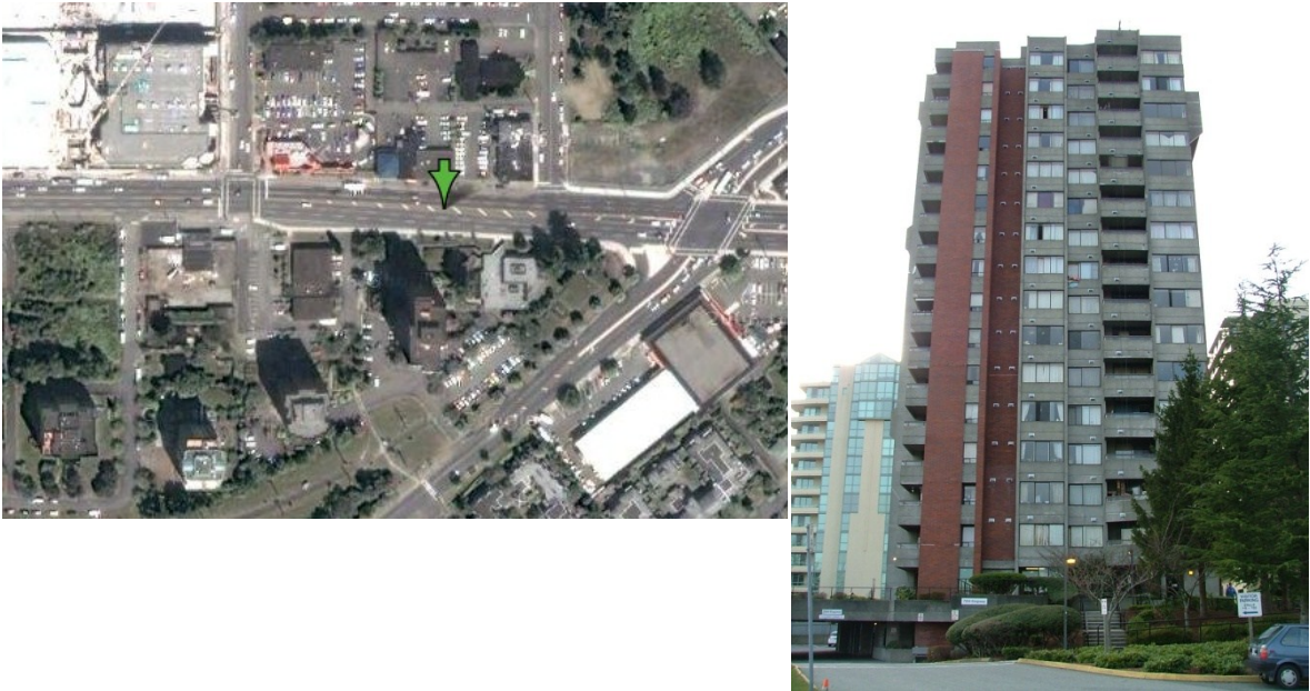
Figure A6.1: Satellite image (left) showing Building 6, which is surrounded by several high-rise buildings to the west and northeast and relatively few obstructions to south, and photograph (right) showing the east exposure of this 16-storey residential building clad with brick veneer and cast-in-place concrete
