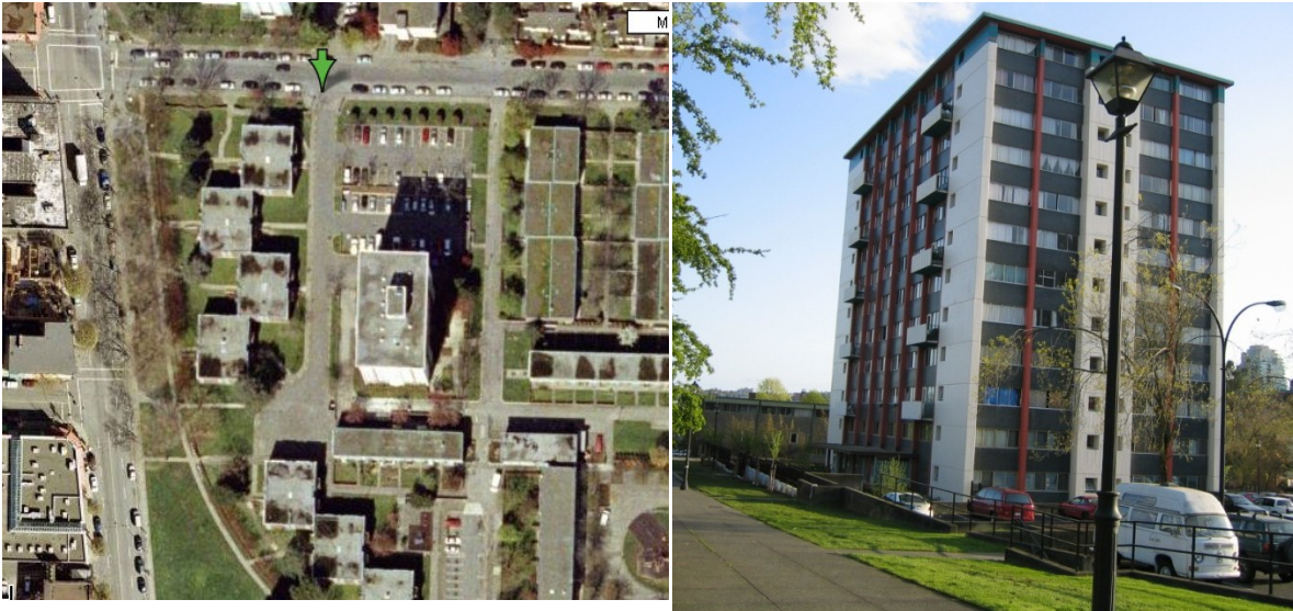
Figure A7.1: Satellite image (left) of Building 7 and its surroundings of low-rise buildings, and photograph (right) showing the 12-storey high-rise residential building with a 3-foot overhang at roof level
