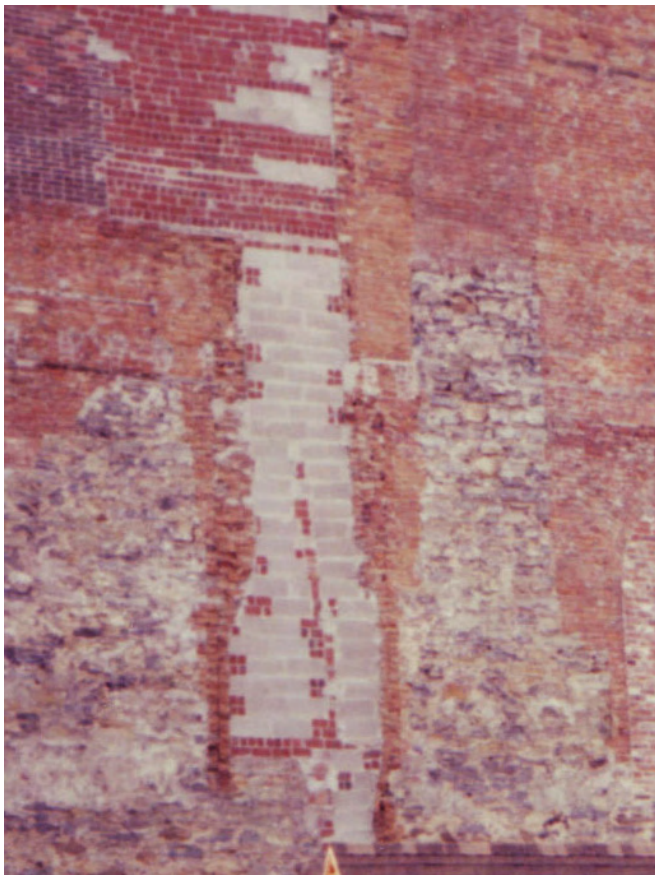
Figure 27: Detail (earlier repairs) of wall on south face of 439-47 St-François-Xavier St., Old Montreal. c 1985, Unknown photographer.
