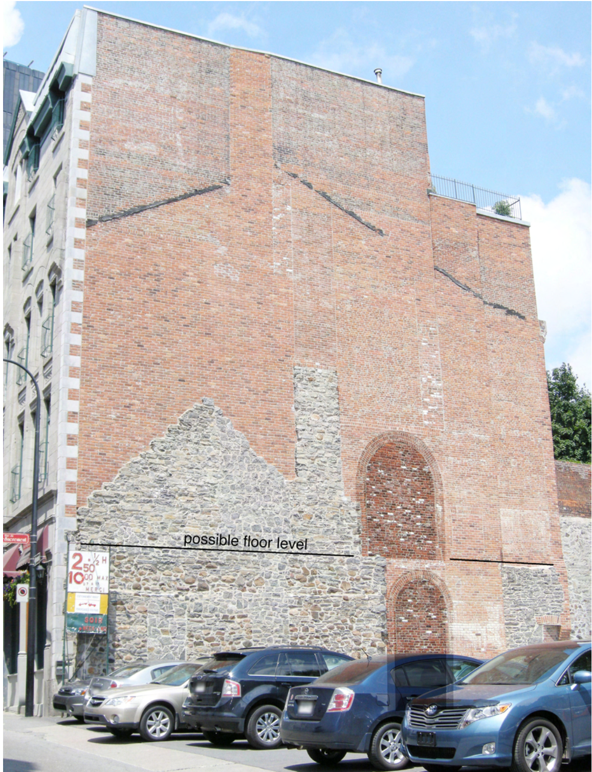
Figure 13: Arched openings and possible second floor ; Wall on south face of 439-47 St-François-Xavier St., Old Montreal. 2010, Personal photograph.
