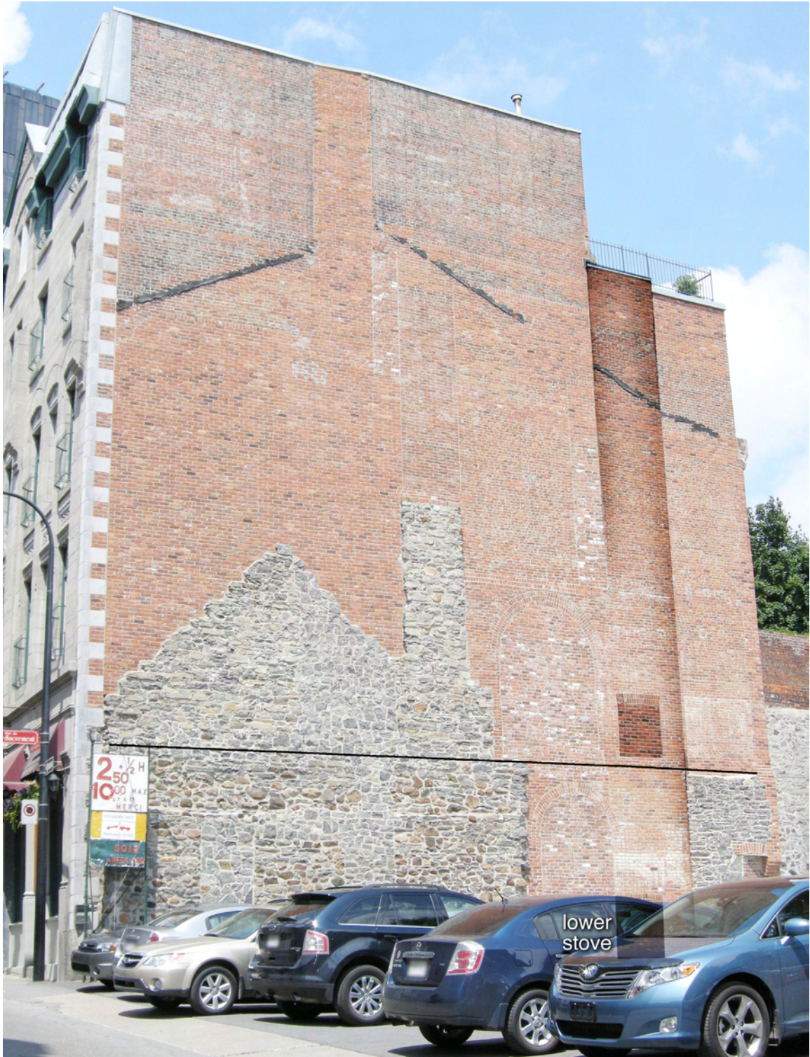
Figure 14: Stoves on two levels and chimney that serves them; Wall on south face of 439-47 St-François-Xavier St., Old Montreal. 2010, Personal photograph.
