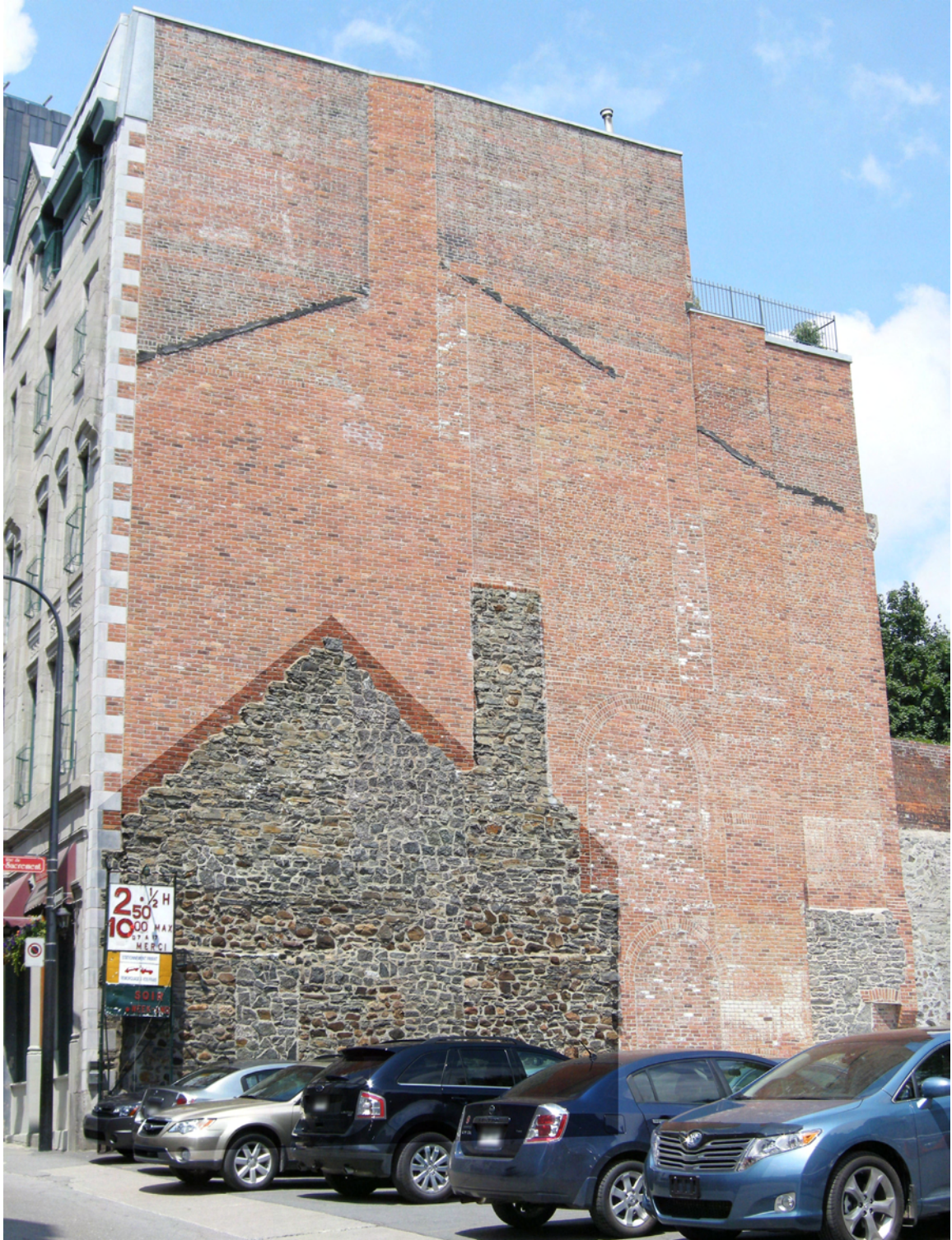
Figure 7: Second house ; Wall on south face of 439-47 St-François-Xavier St., Old Montreal. 2010, Personal photograph.
