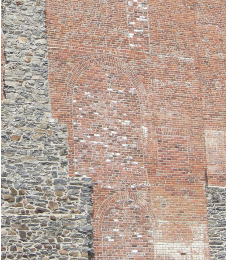
Figure 5: Detail of wall on south face of 439-47 St-François-Xavier St., Old Montreal. 2010, Personal photograph.
