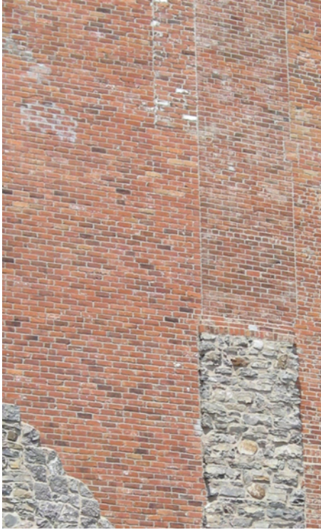
Figure 10: Detail of chimney definition on wall on south face of 439-47 St-François-Xavier St., Old Montreal. 2010, Personal photograph.
