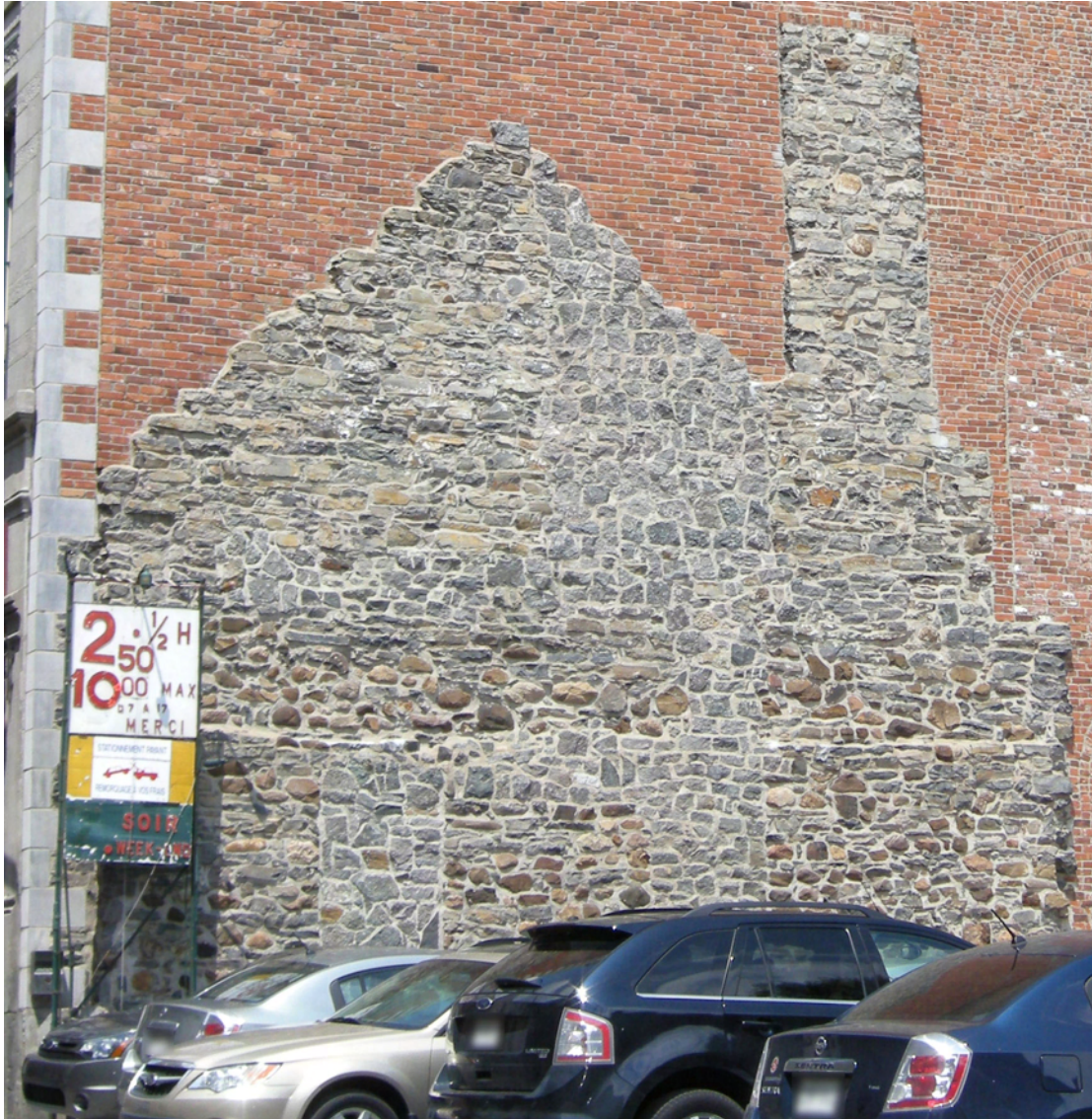
Figure 4: Detail of wall on south face of 439-47 St-François-Xavier St., Old Montreal. 2010, Personal photograph.
