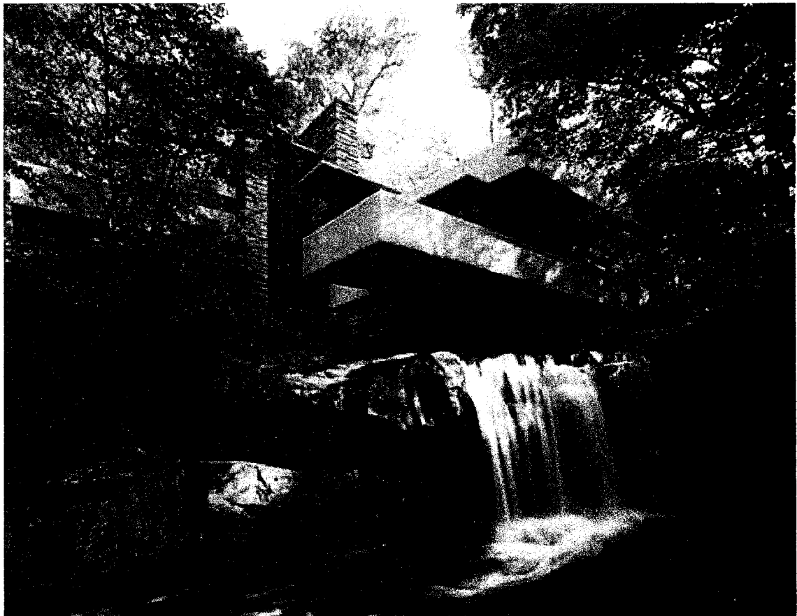
Fig. 35 Frank Lloyd Wright, Fallingwater (1934) Bear Run, Pennsylvania
