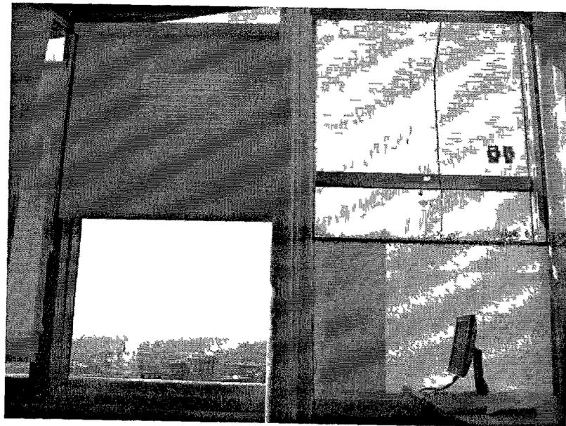
*Figure 1 1 Comparison of a conventional roller shade (on the left) with a bottom-up roller shade (on the right), emphasizing the operational direction*
