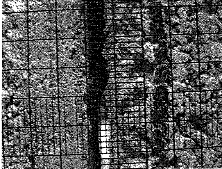
Figure 4.1 Observed head joint crack located at the constant moment zone of a specimen
