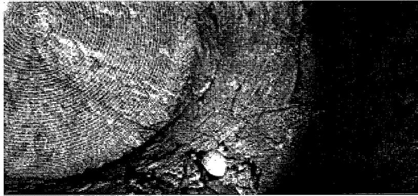
**Figure 2-12 Grooves of disc cutter on hard rock tunnel face by a TBM machine (Herrenknecht, 2008).**
