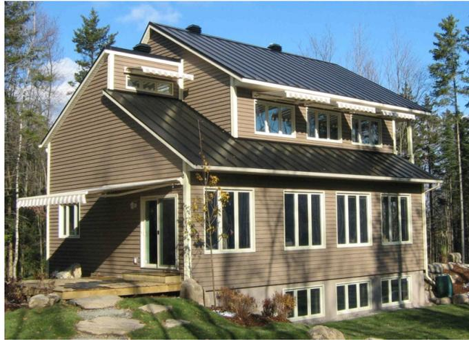
Fig. 1.4: ÉcoTerra demonstration house, November 2007 (the photovoltaic system made up of amorphous Silicon laminate panels attached to metal roof is on the upper roof section).
