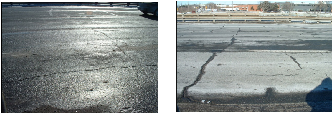
Figure 31: Surface Cracks on the Asphalt Wearing Surface (Courtesy of MTO 2003)
