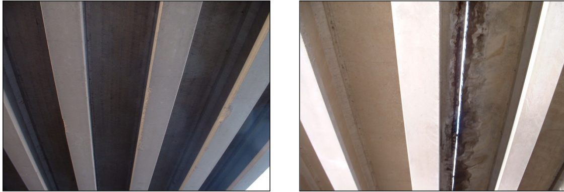
Figure 32: Typical Condition of Deck Soffit (Courtesy of MTO 2003)
