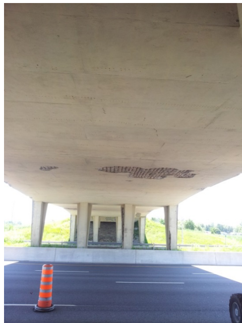
Figure 28: Localized Scaling Area on the Deck Soffit (Photo Courtesy of Sami Moufti 2013)
