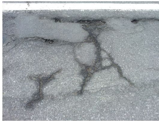
Figure 27: Deterioration of Deck Wearing Surface (Photo Courtesy of Sami Moufti 2013)
