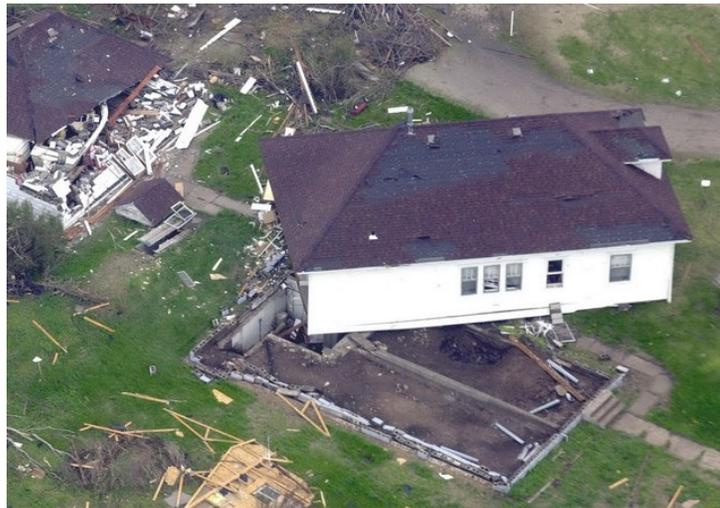
Figure 1.1: Low-rise building damage likely caused by wind-induced torsion (AAWE, 2013)
