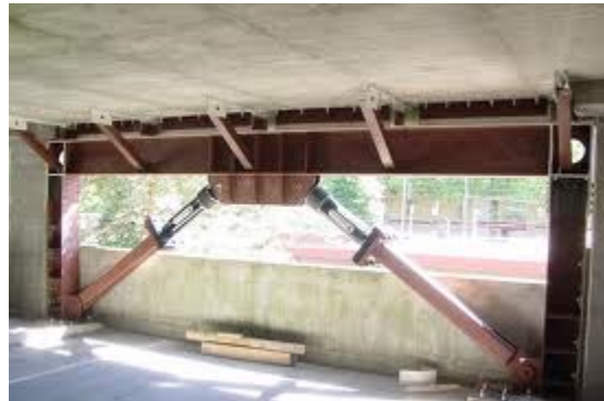
Figure 2-11: Viscous fluid damper installation arrangement (Symans et al, 2008)
