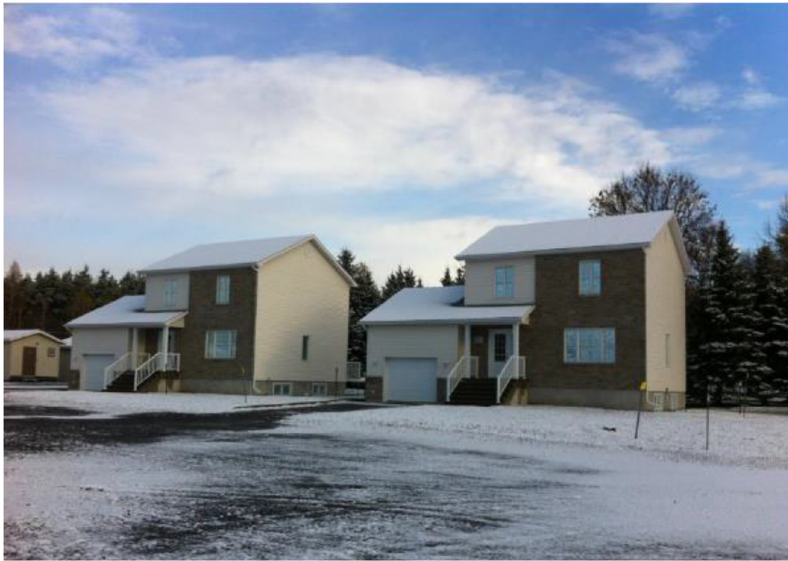
Figure 4.39. Twin houses test facility in Shawinigan (Photo courtesy of Jennifer Date)
