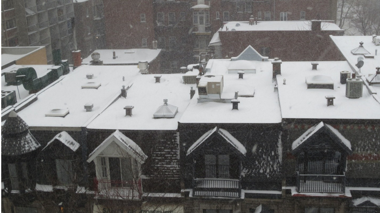
Figure 2-6. Snow cover on a residential building roof during the winter in Montreal.
