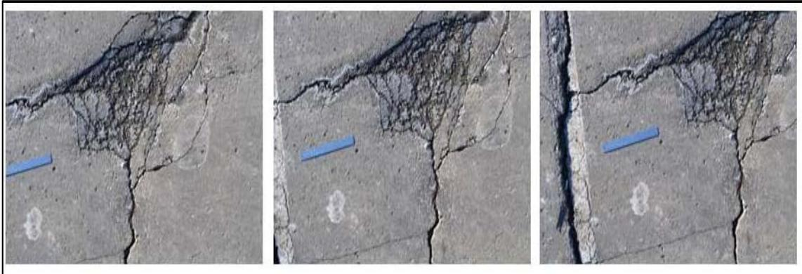
Figure 2-11 3DOBS application in calculating the surface defects (Ahlborn et al. 2013)
